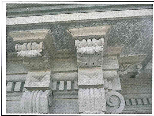
Process of honing the soffit
