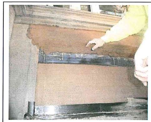
Starting to install the repair
