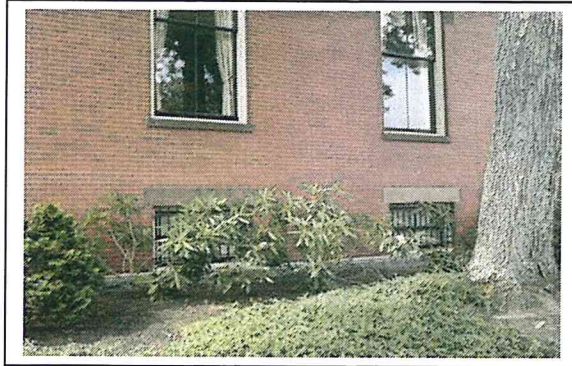
Basement lintels use salvaged stone
