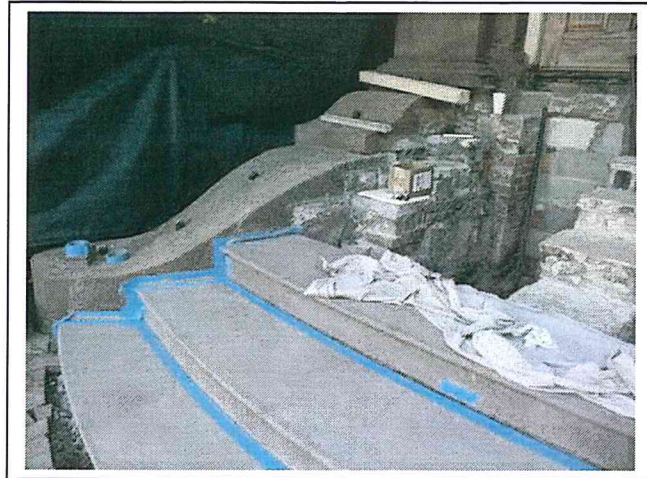
Installation of new steps
