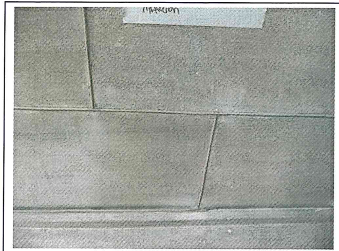
Mock-ups for repointing
