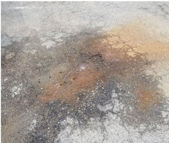
Examples of the driveway damage caused by water overflow from the drainage swale as a result of the Phragmites
