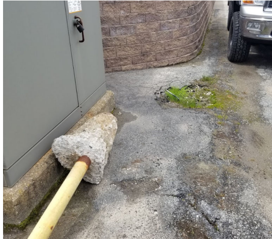
Examples of the driveway damage caused by water overflow from the drainage swale as a result of the Phragmites
