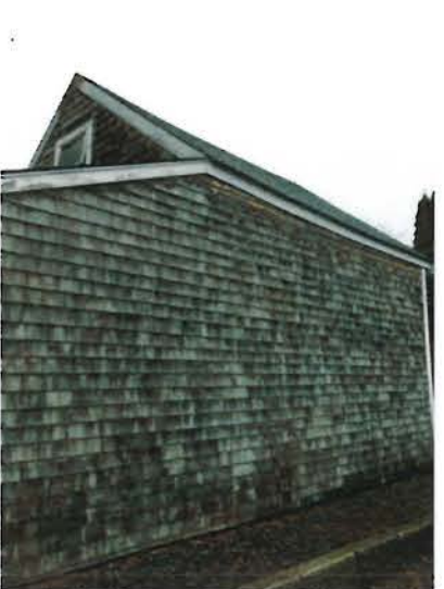
7 View of East Elevation
