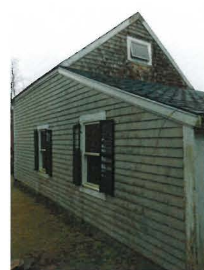
3 View of West Elevation
