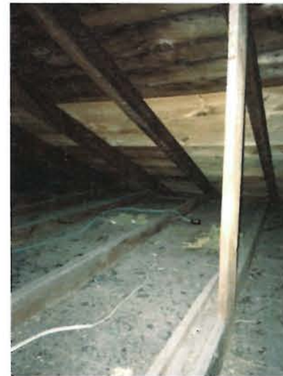
1 View of Attic Framing
