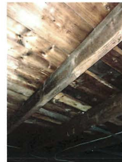
5 View of Loft Framing
