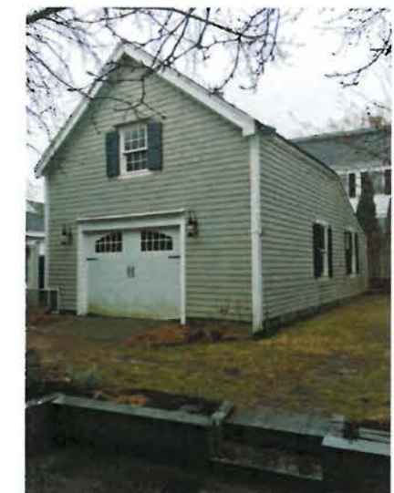
4 View of North Elevation
