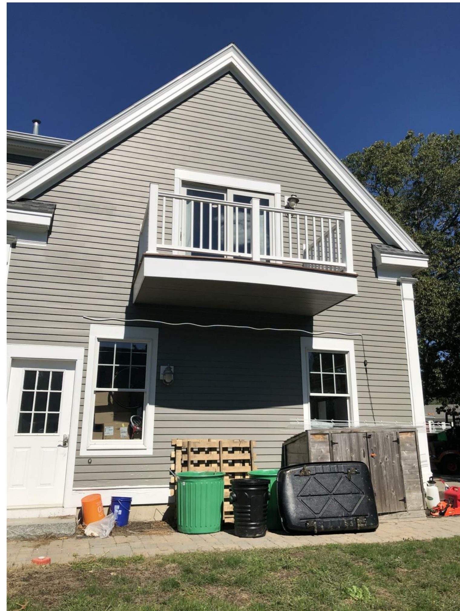
4 EXISTING CONDITIONS IMAGE OF SOUTHEASTERN FACADE
