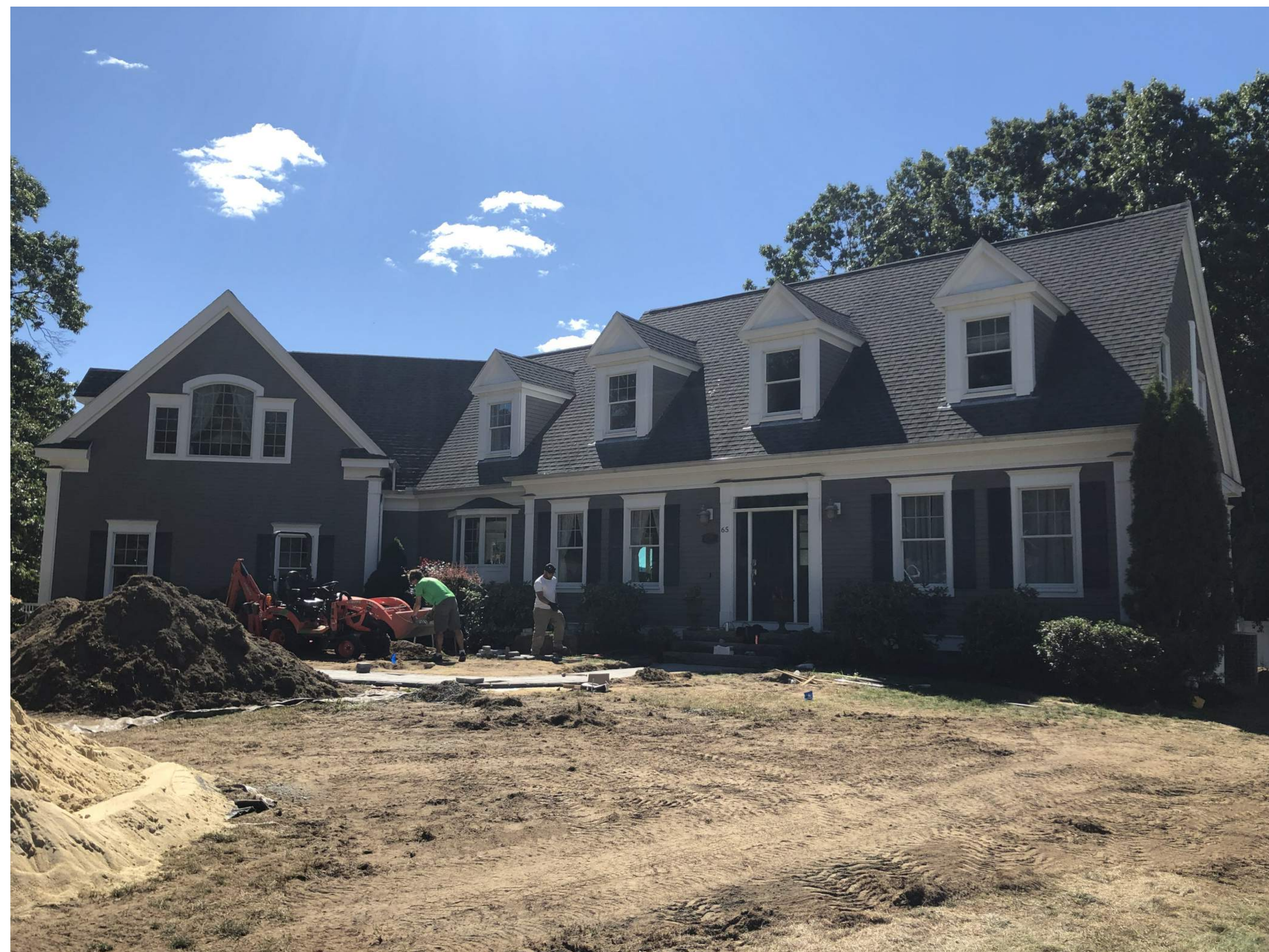
1 EXISTING CONDITIONS IMAGE OF NORTHEAST FACADE
