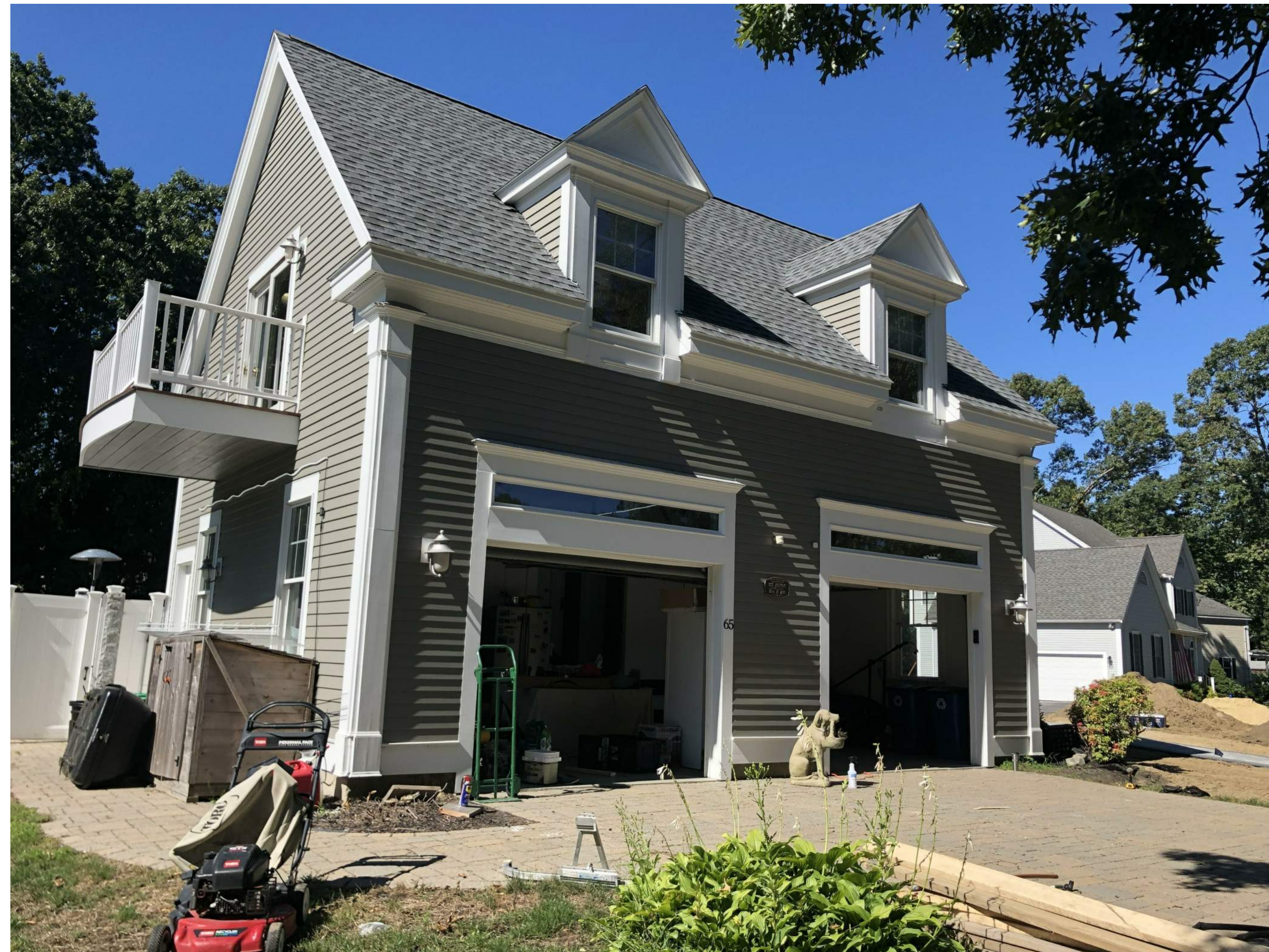
3 EXISTING CONDITIONS IMAGE OF SOUTH CORNER 1/2" = 1'-0"
