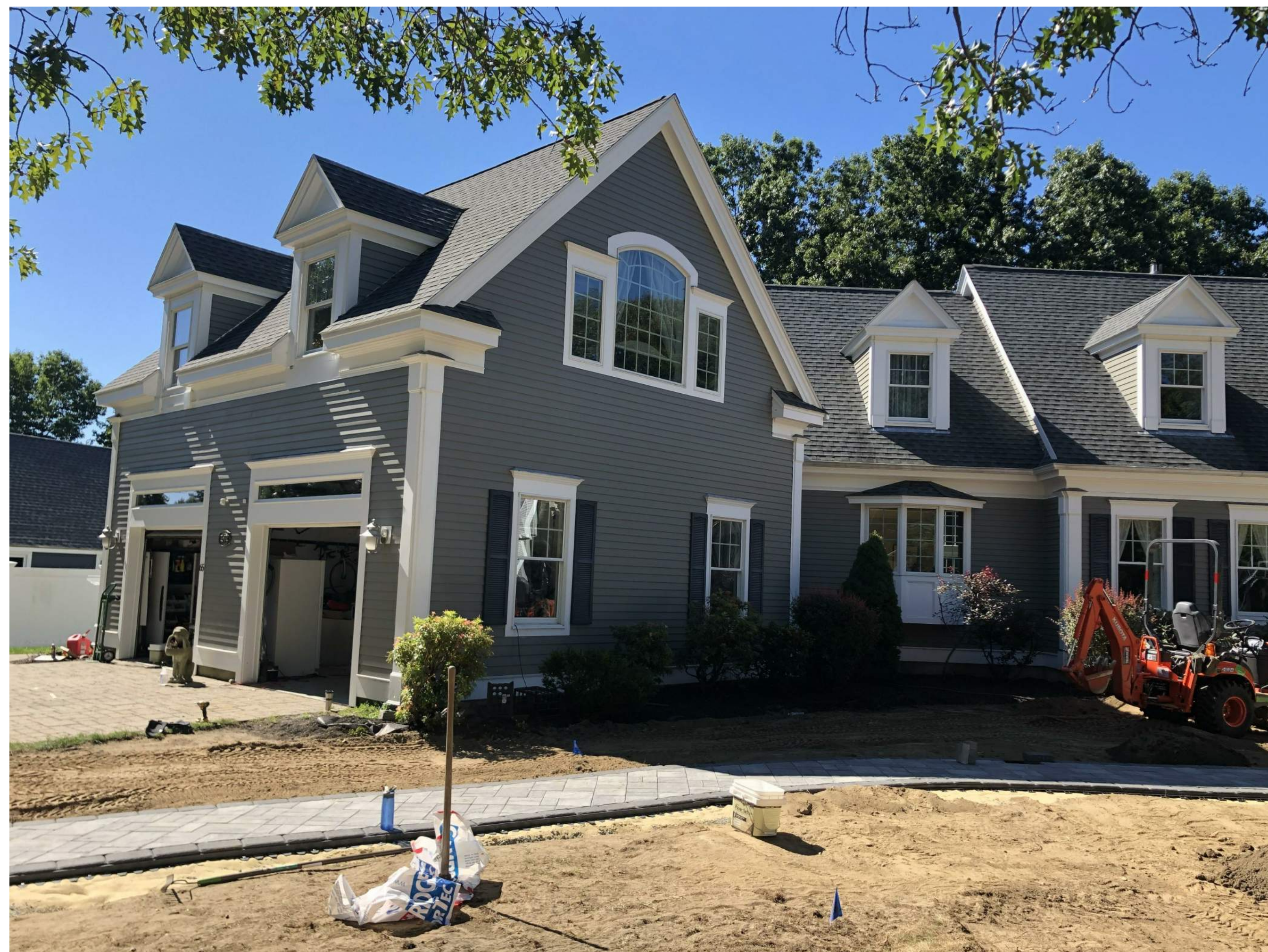
2 EXISTING CONDITIONS IMAGE OF EAST CORNER
