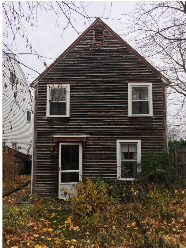
1 View from Rear Yard
