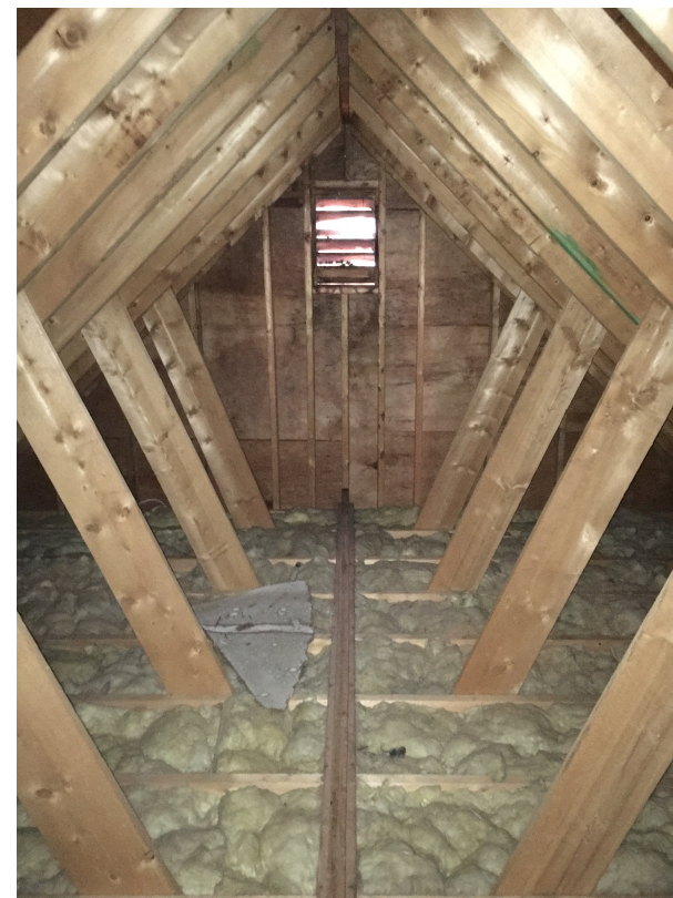
6 Circa 1980 Attic Framing
