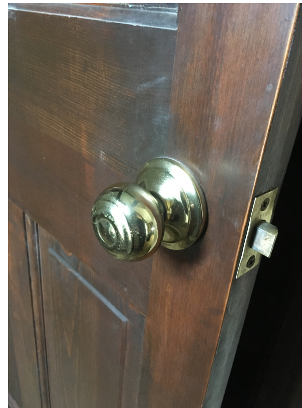
7 Typical Interior Door
