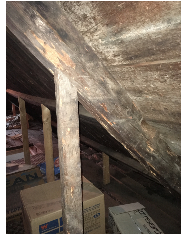
4 Circa 1800 Attic Framing
