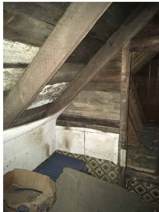
5 Circa 1930 Attic Framing
