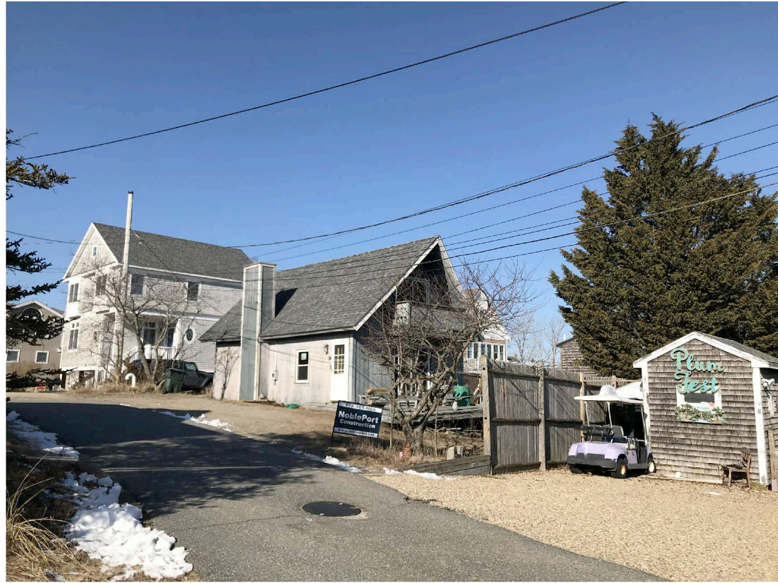
VIEW FROM INTERSECTION OF 68th + NORTHERN BLVD
