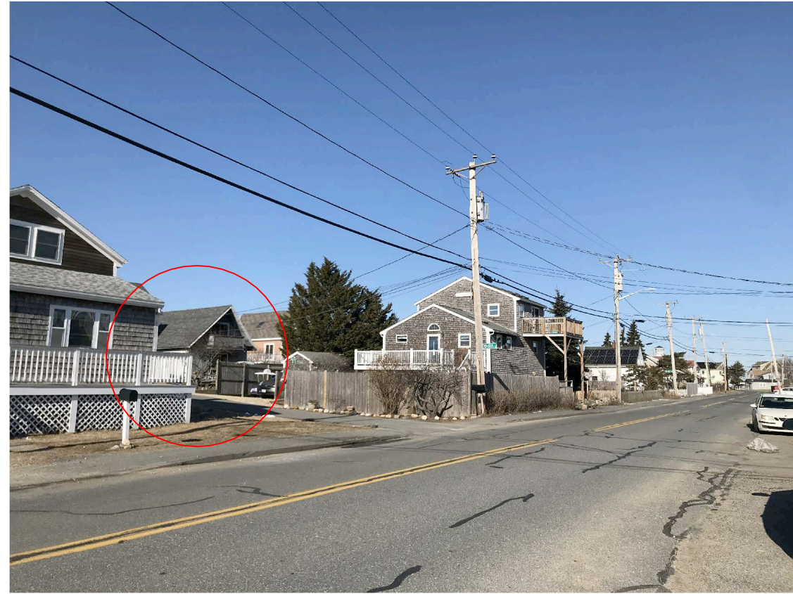
VIEW FROM NORTHERN BLVD
