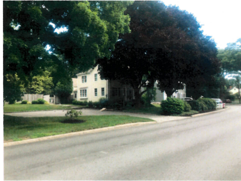
42 TOPPANS LANE 2 Houses to Right
