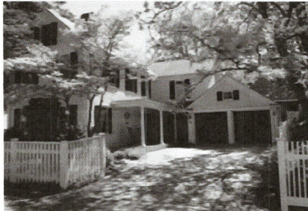
40 Middle Street - Existing View from the Street
