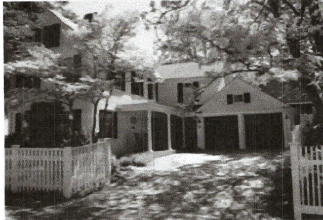
40 Middle Street - Existing View from the Street
