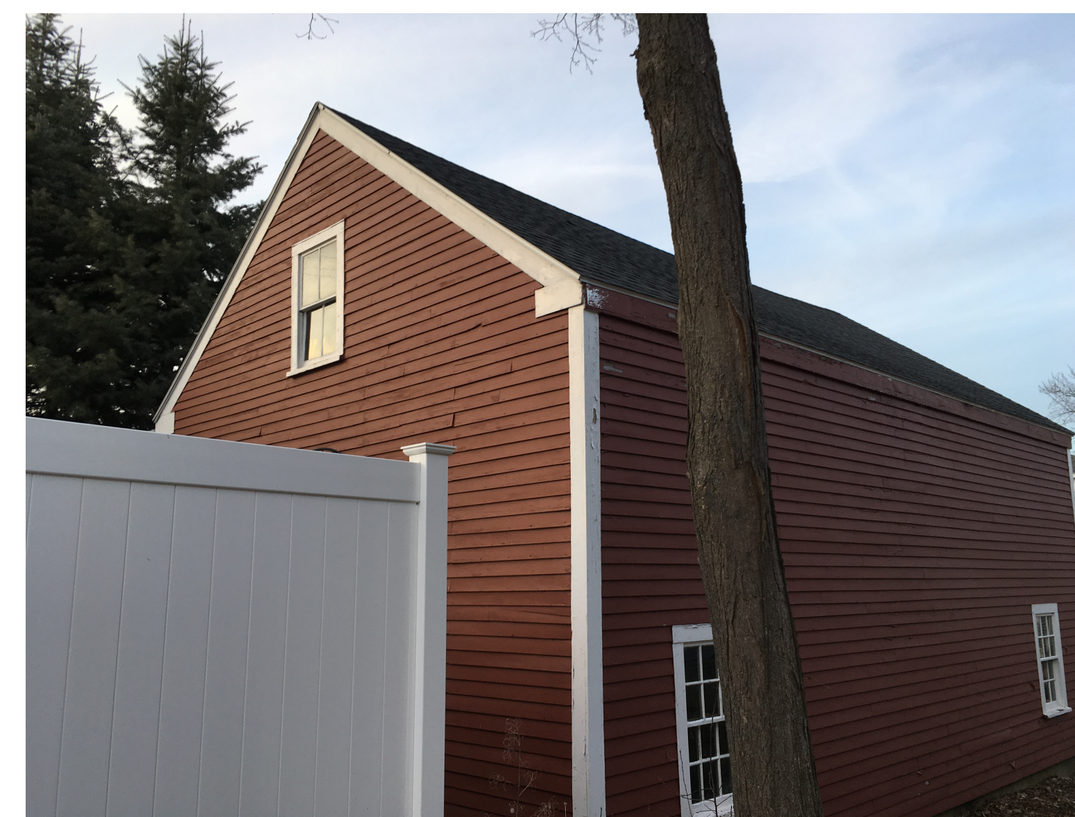
EXISTING - BARN REAR / RIGHT
