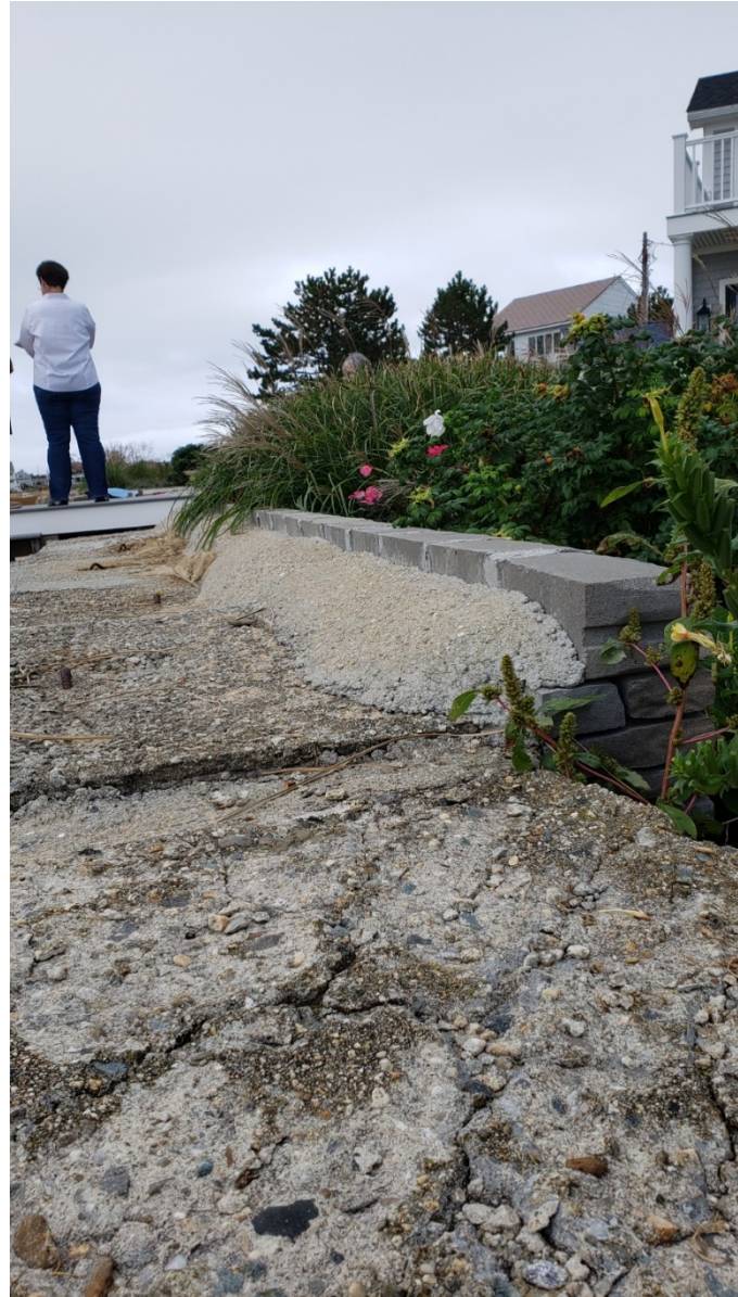
The above two photos show the top of one section of the stone facing connected to the blocks by a line of concrete.
