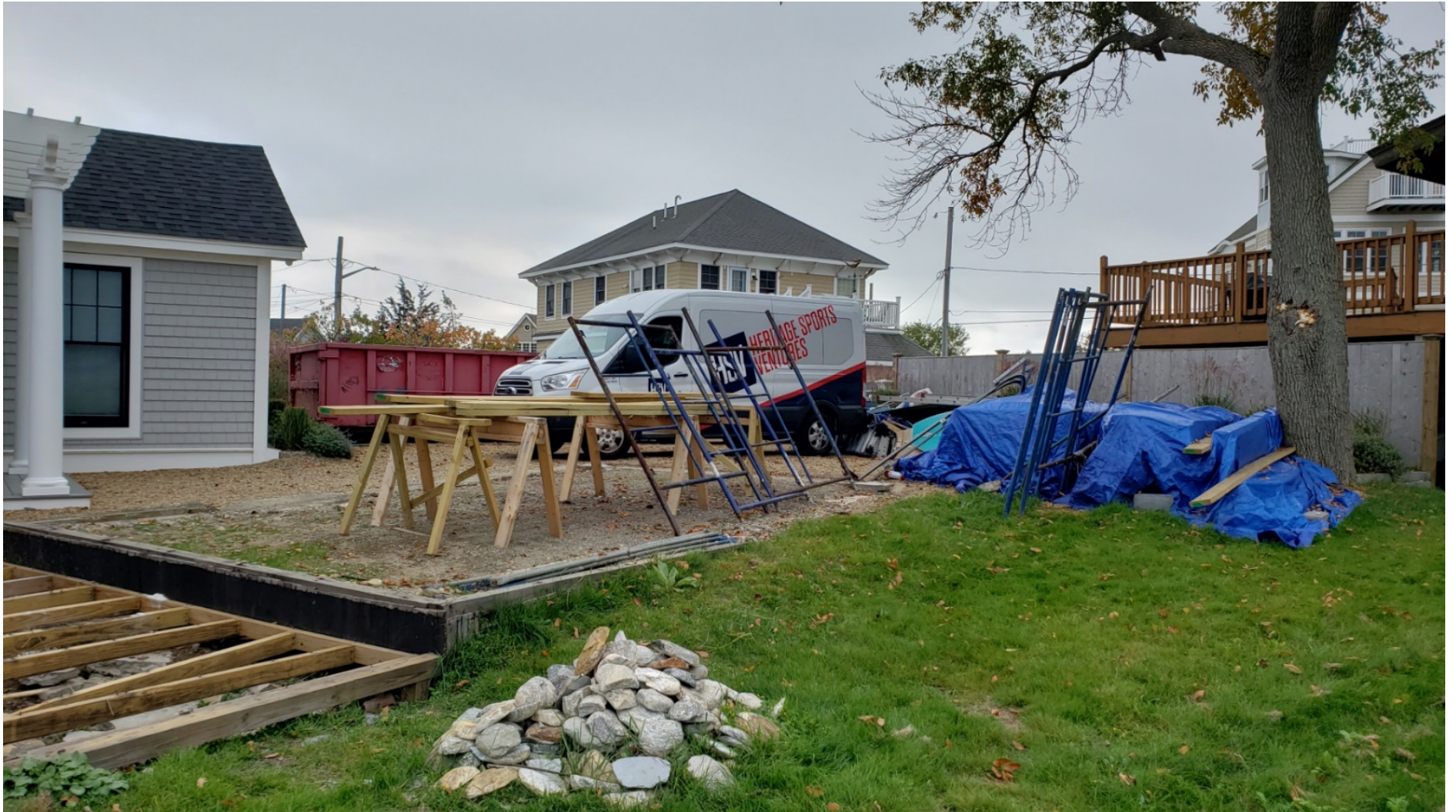
The above photo shows the demolished garage foundation.
