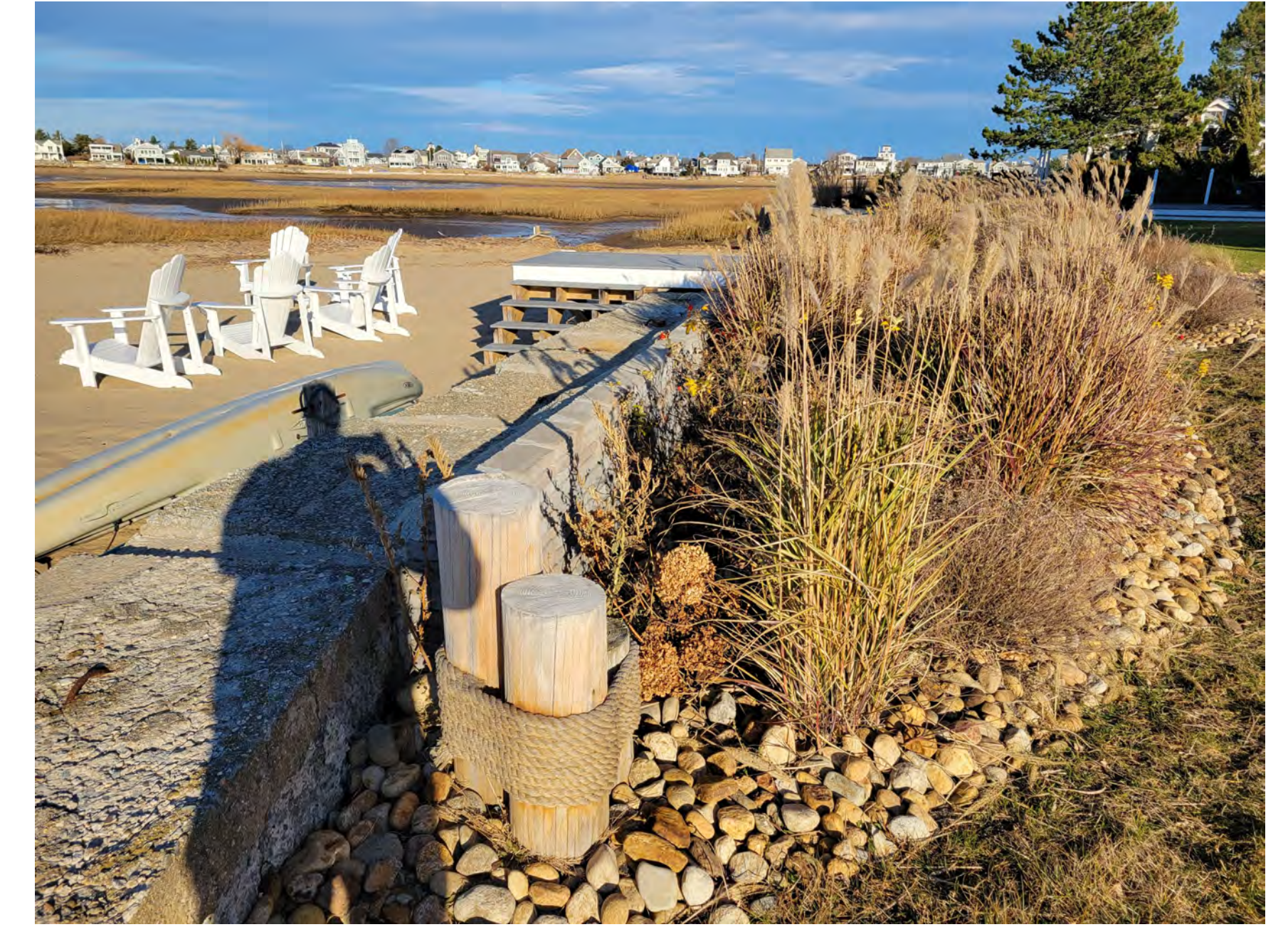
Replaced stairs on left, typical planting bed on right
