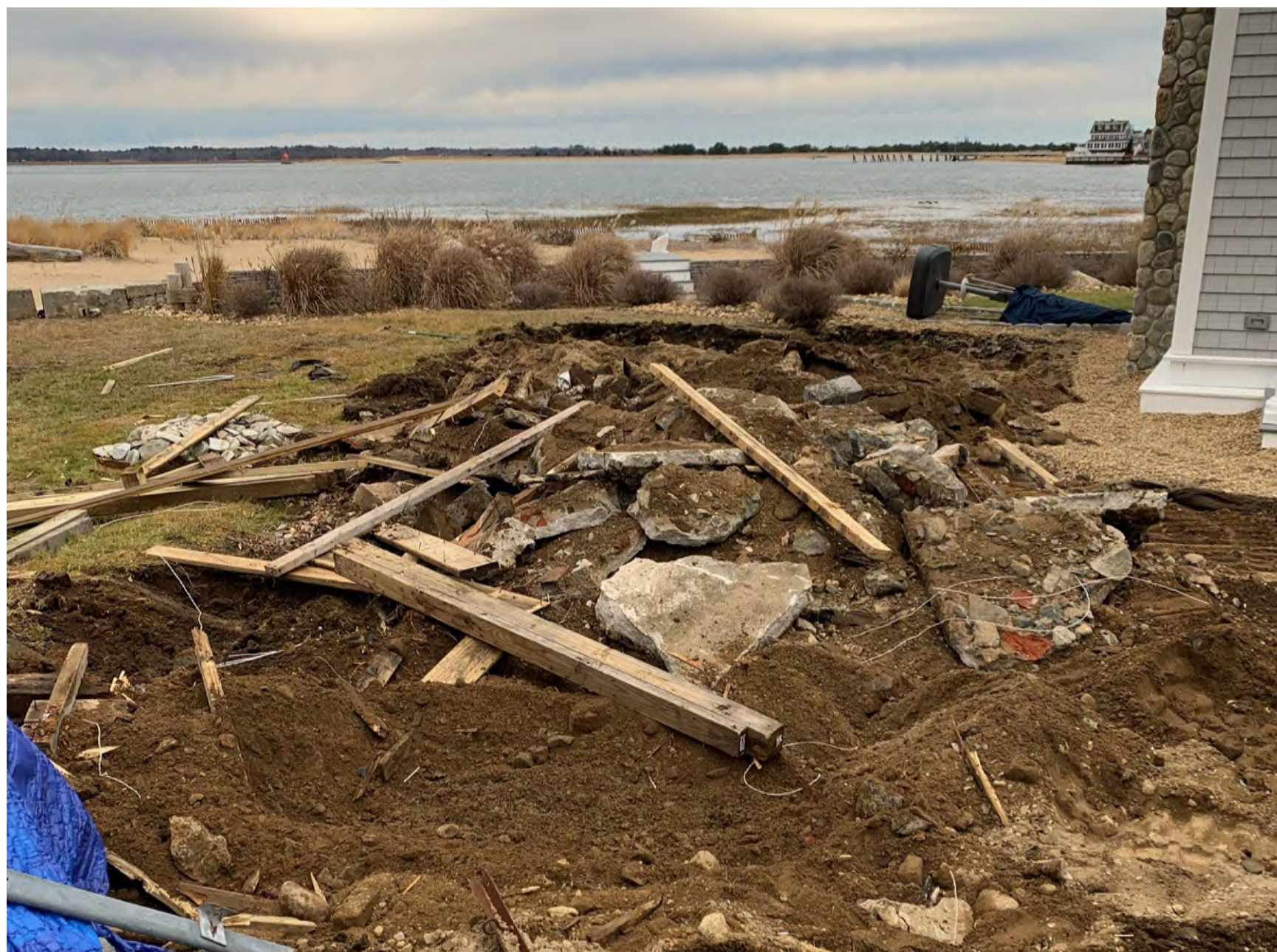
Concrete and platform being removed
