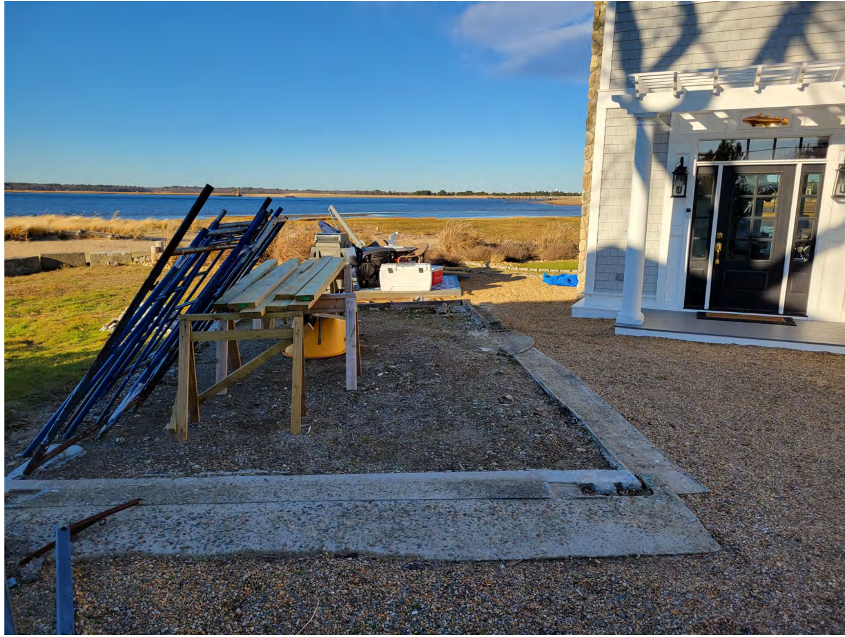
Area of old garage, concrete extends towards house
