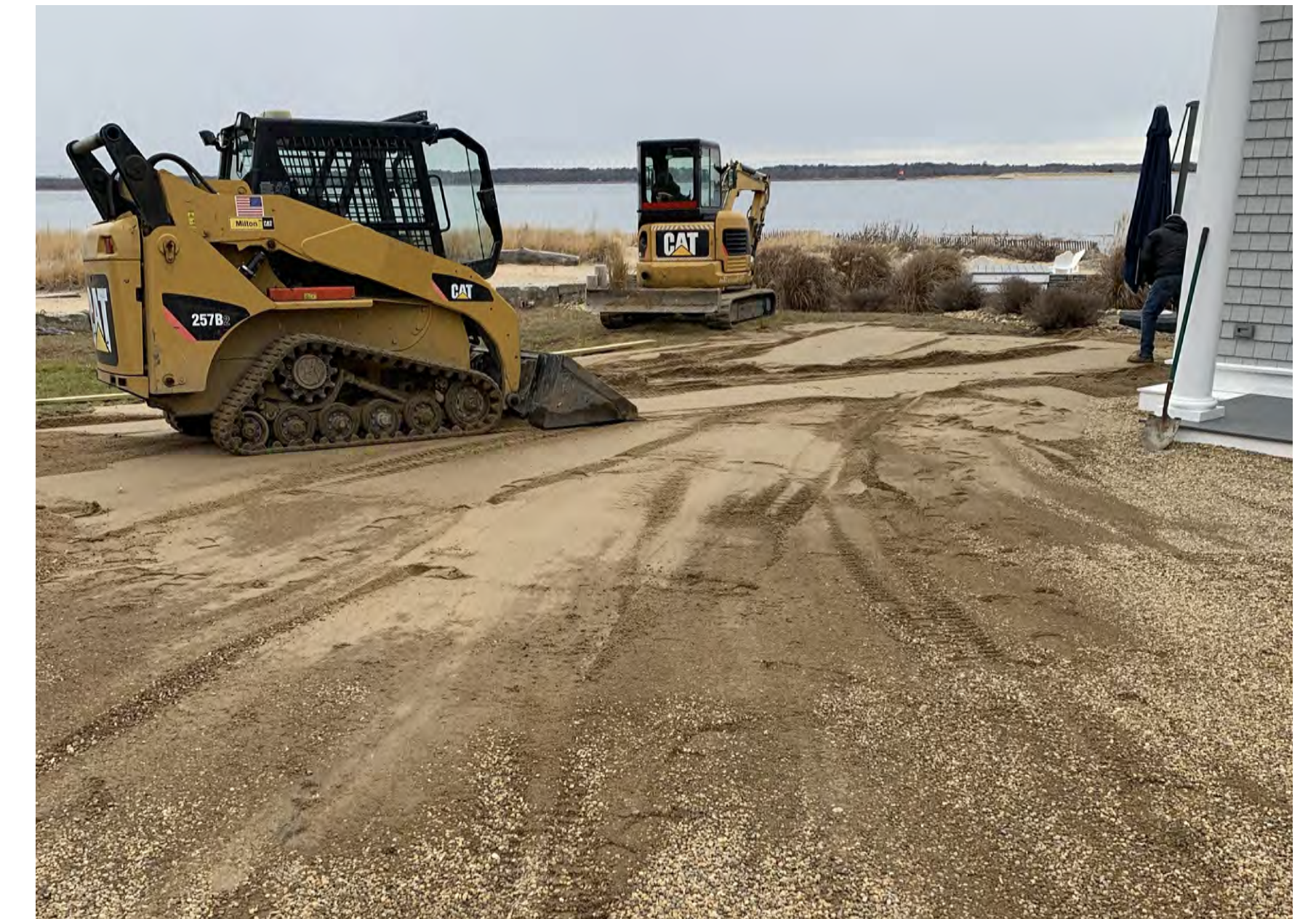
Area backfilled with clean sand
