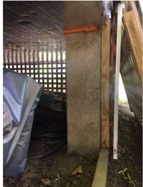
Sunroom existing concrete footing
