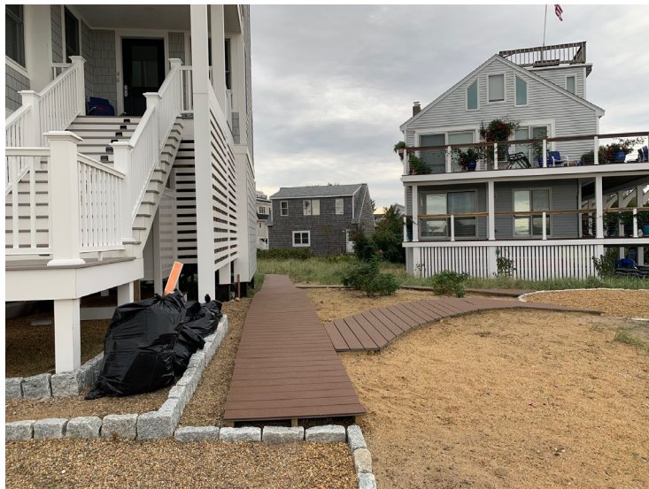
Photo 4: View on west side of house from Reservation Terrace
