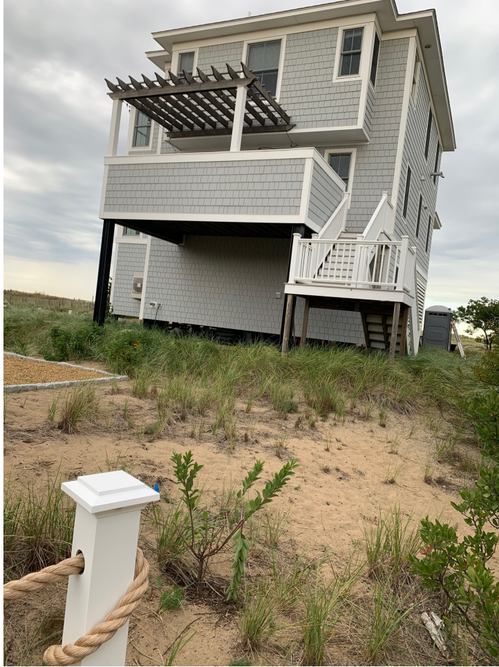
Photo 1: Rear (south) view from 65 th Street
