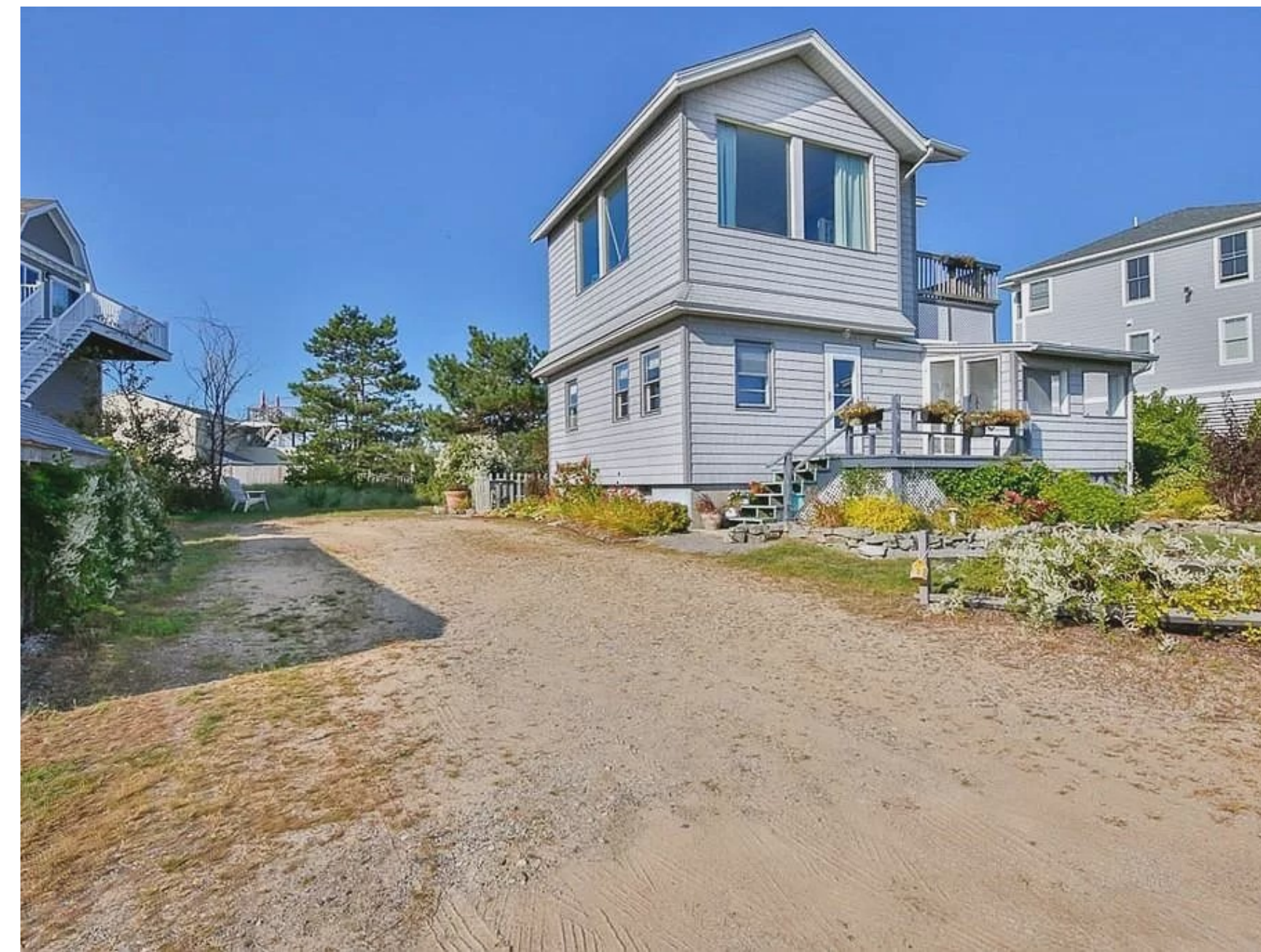
Existing Gravel Drive
