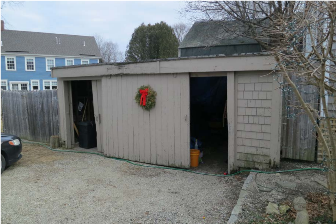
30_View southeast showing northwest elevation of shed
