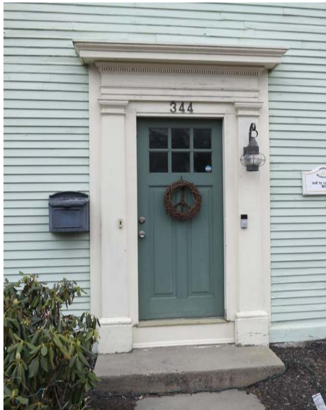
9_View northeast showing principal facade (northwest elevation) - detail of main entry
