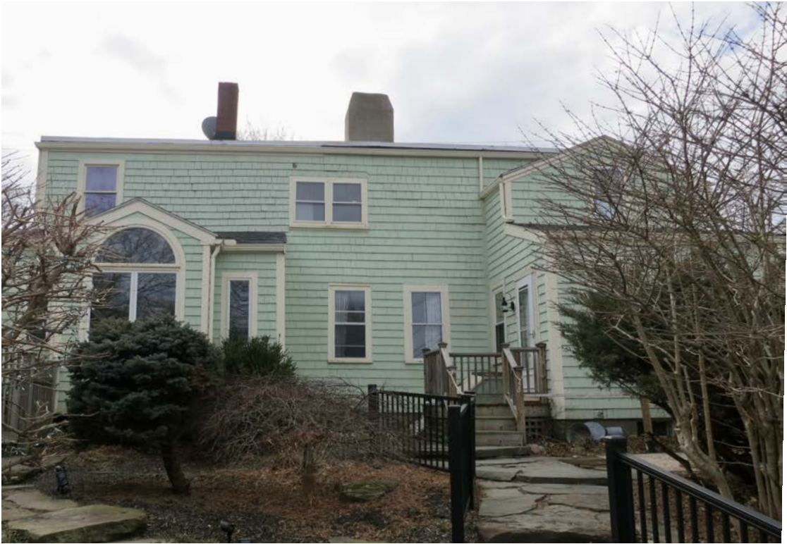
22_View southwest showing rear (southeast) elevation
