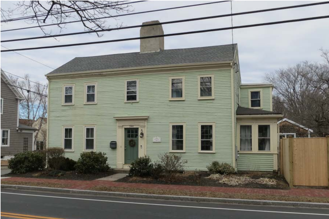
5_ View northeast showing principal facade (southwest elevation)
