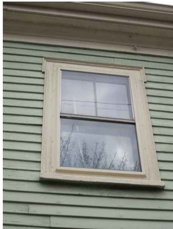
11_View northeast showing principal facade (northwest elevation) - detail of second floor window at south end
