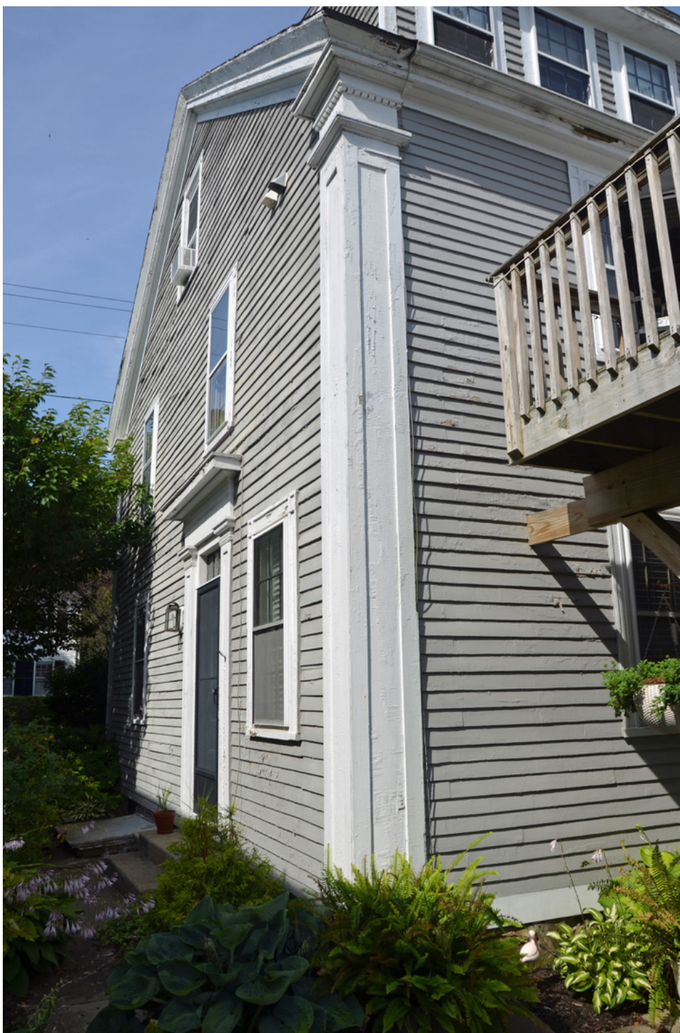
12. Corner Pilaster, Rake, Fascia and Return Detail
