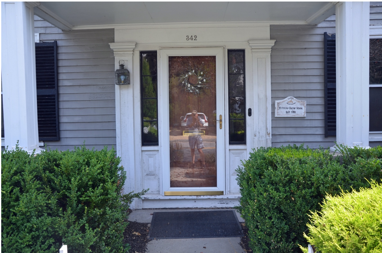
2. Front Entry, Sidelights, Panels, and Pilasters
