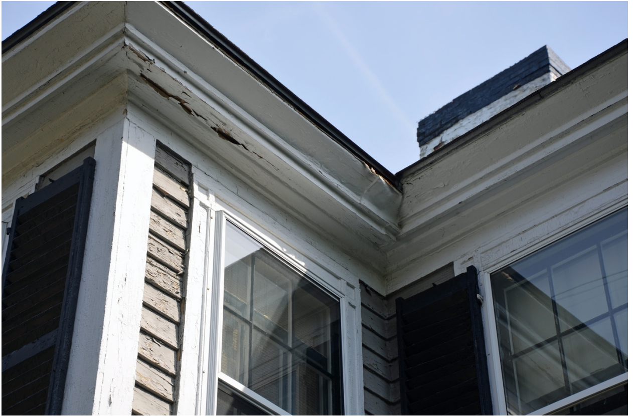
5. Fascia, Crown, Soffit, Frieze and Casing Detail
