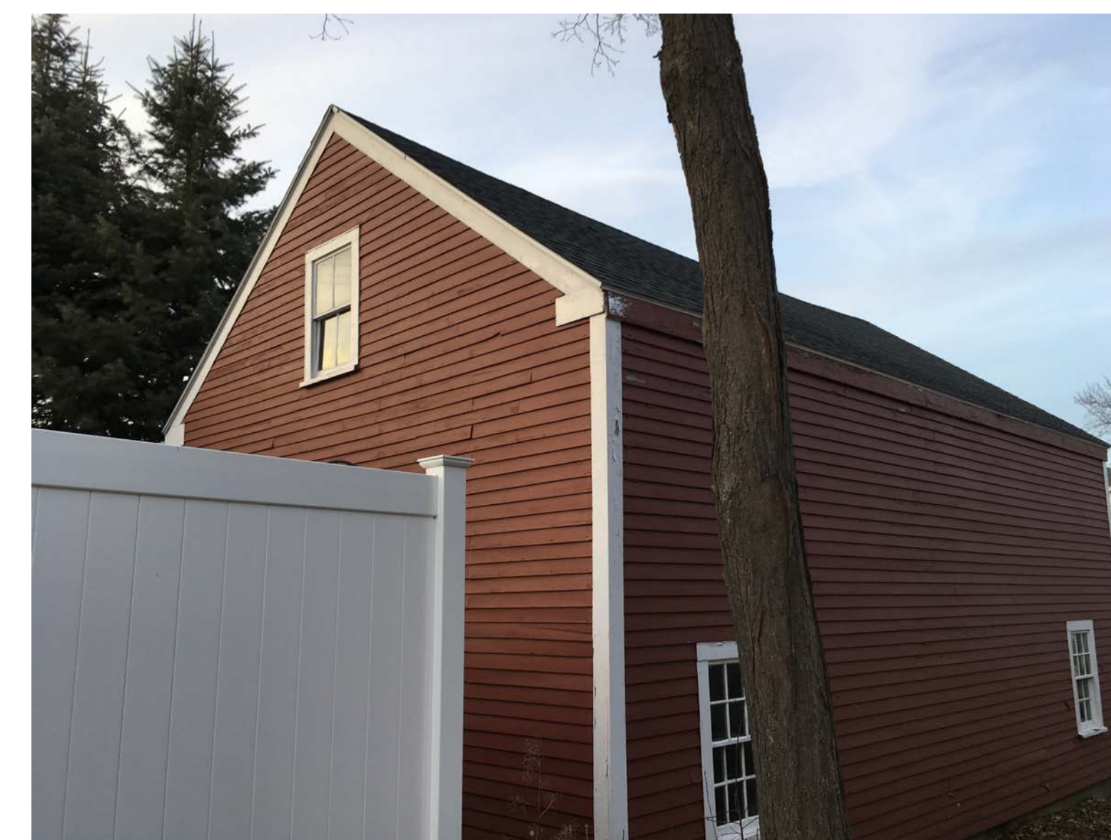
EXISTING - BARN REAR / RIGHT
