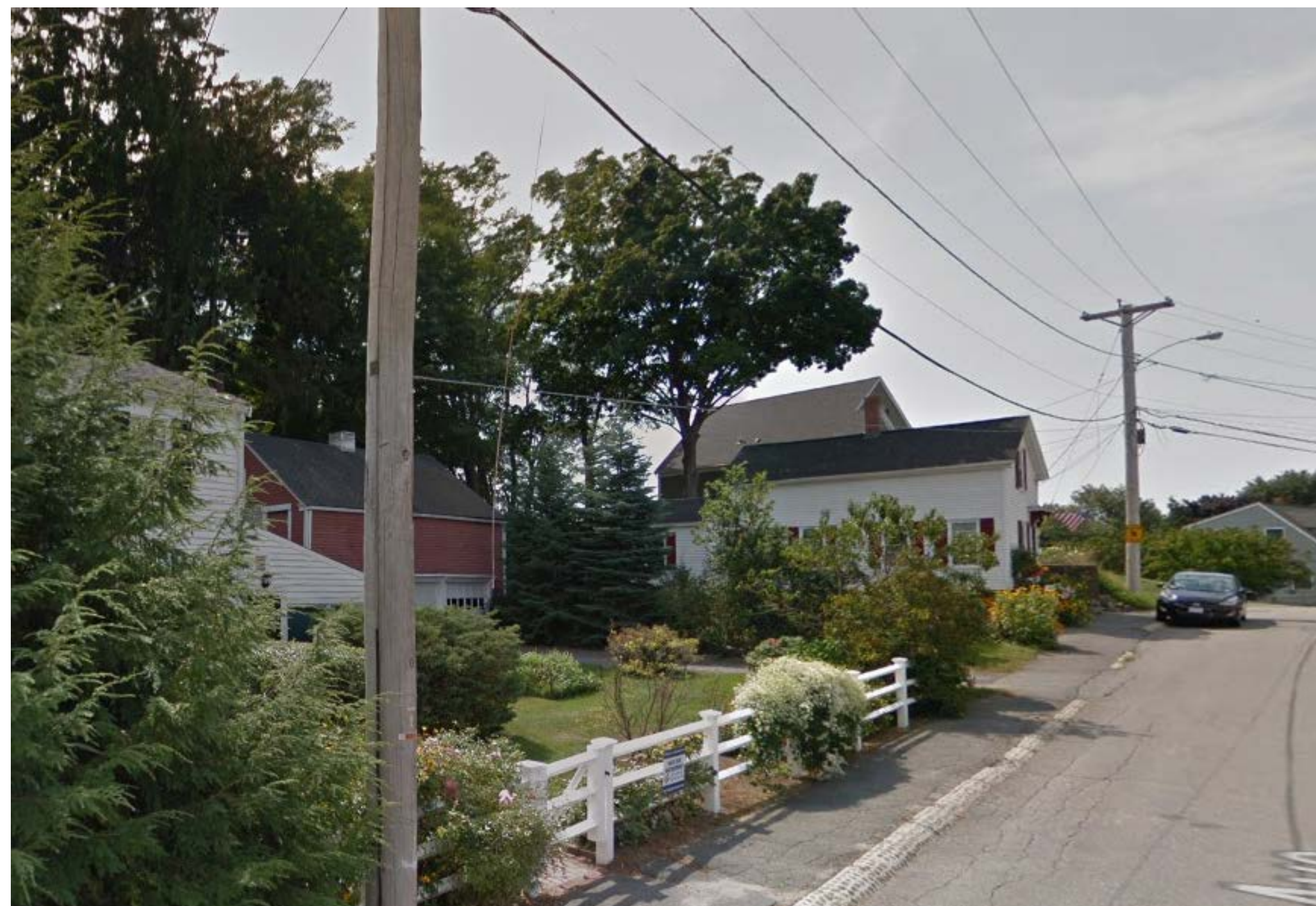
EXISTING - BARN STREET VIEW
