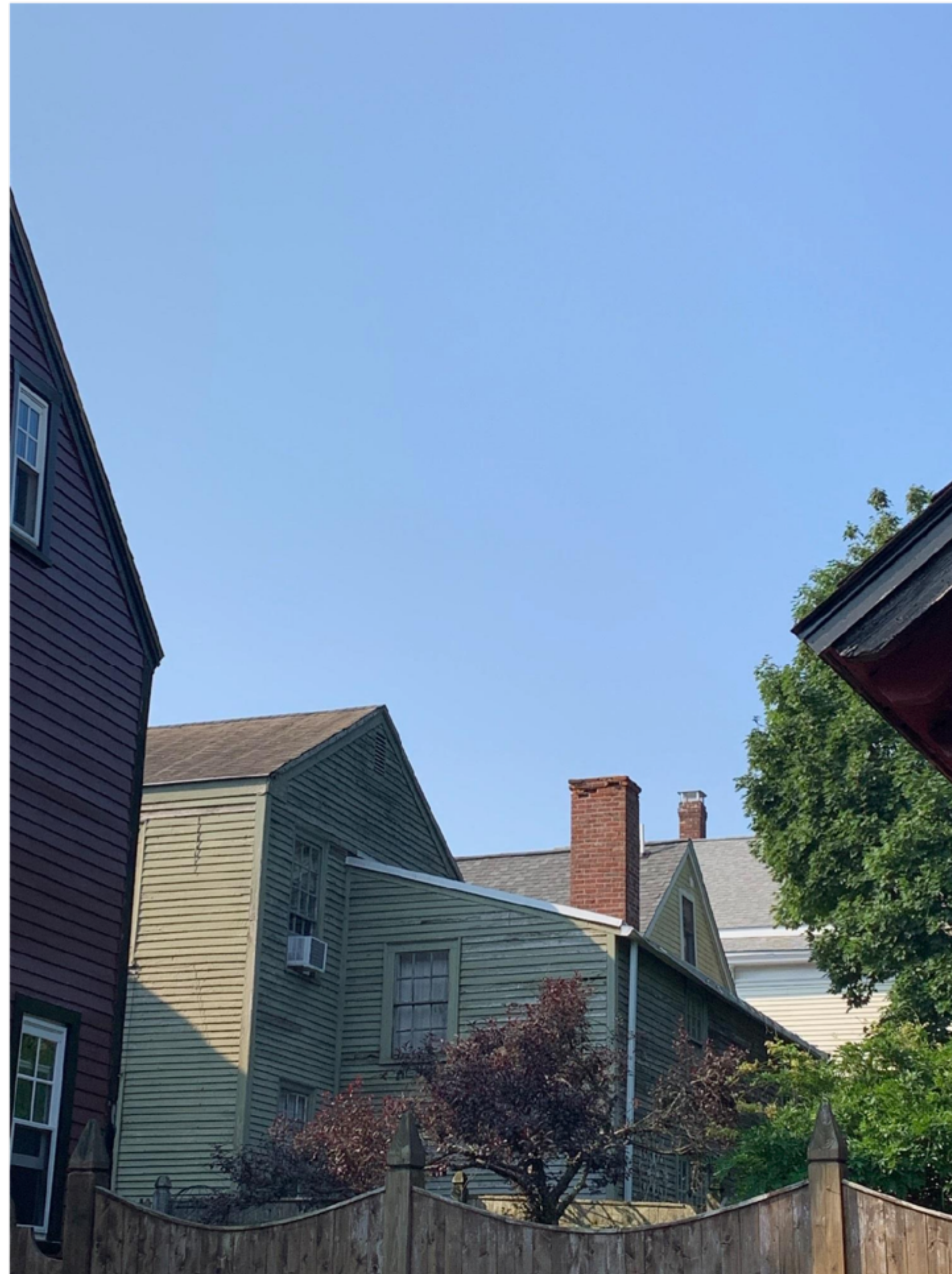
Rear right side looking from Washington St
