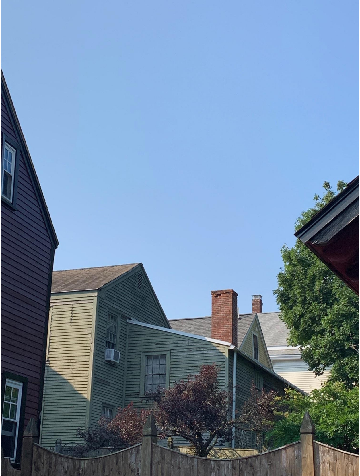
Rear right side looking from Washington St
