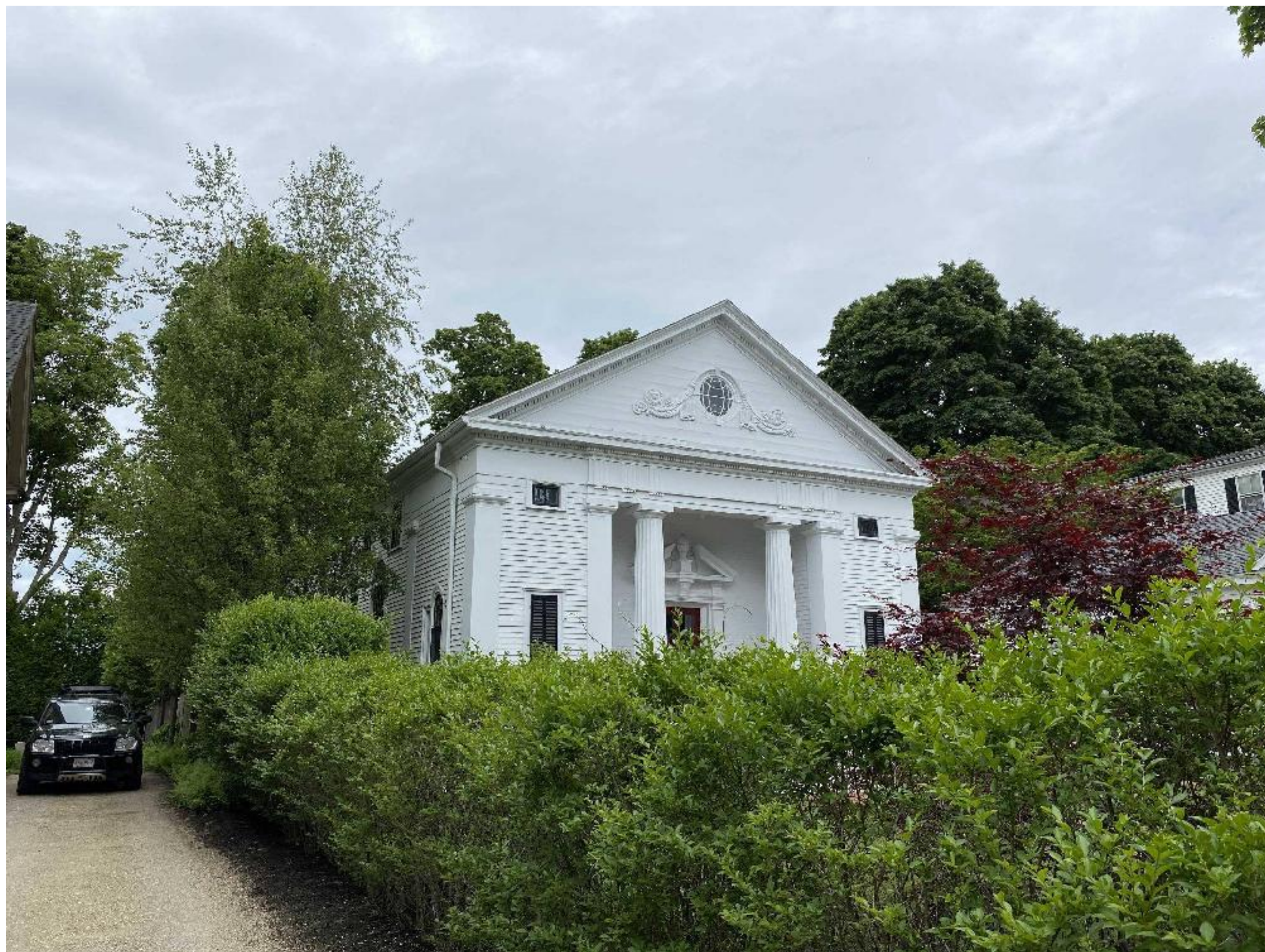
1 EXISTING NORTH-WEST CORNER
