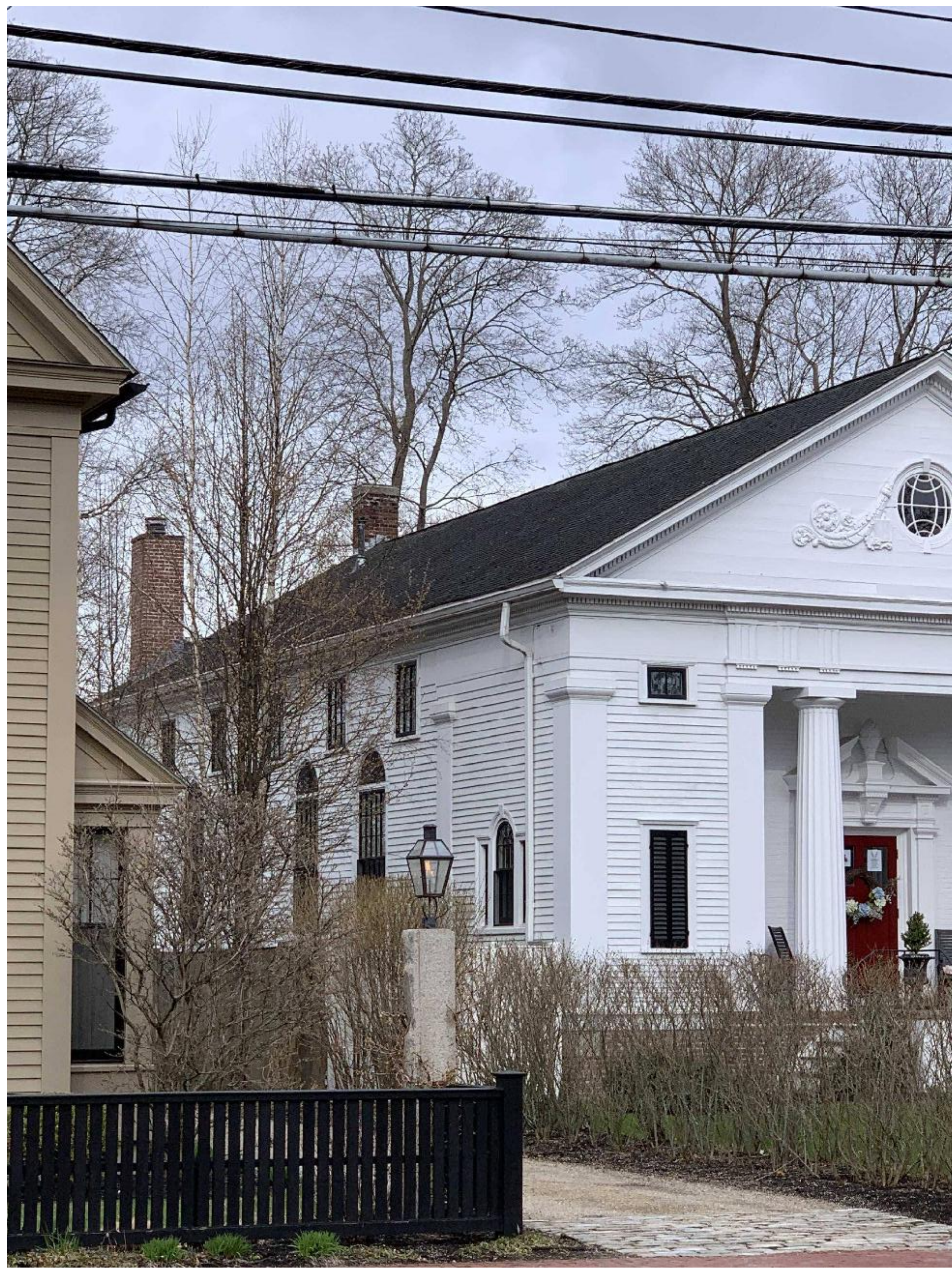
1 EXISTING NORTH-WEST CORNER
