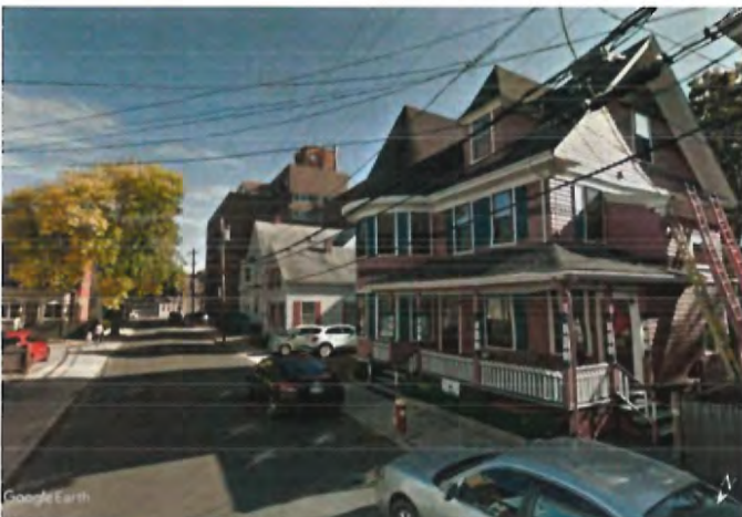
View of the host structure and surrounding area facing southeast.
