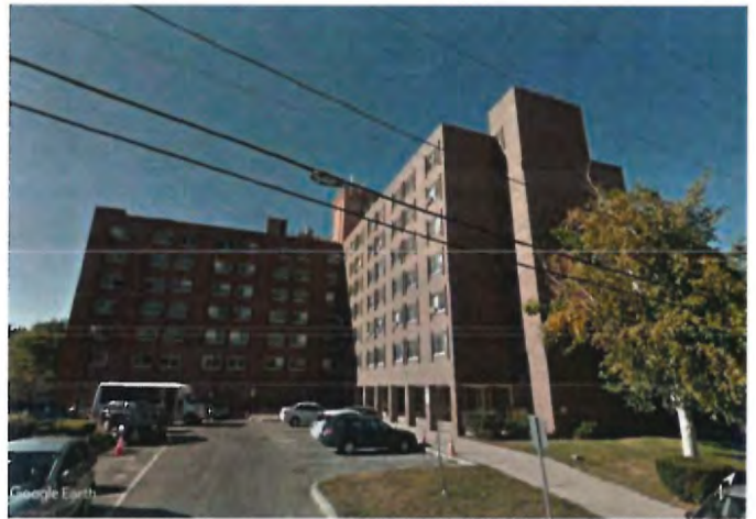
View of the host structure facing northwest.
