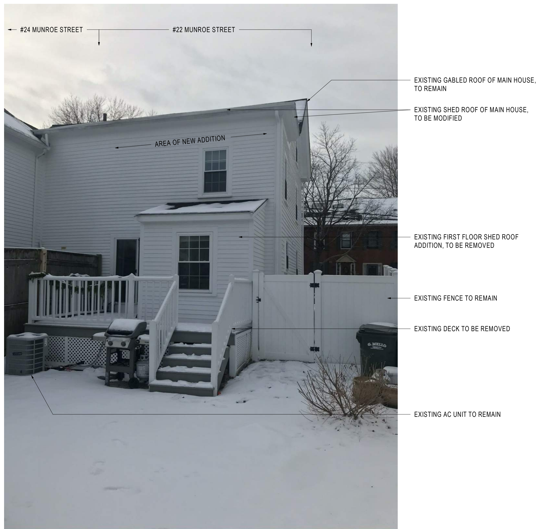
BACKYARD OF 22 MUNROE (NORTH FACADE)
