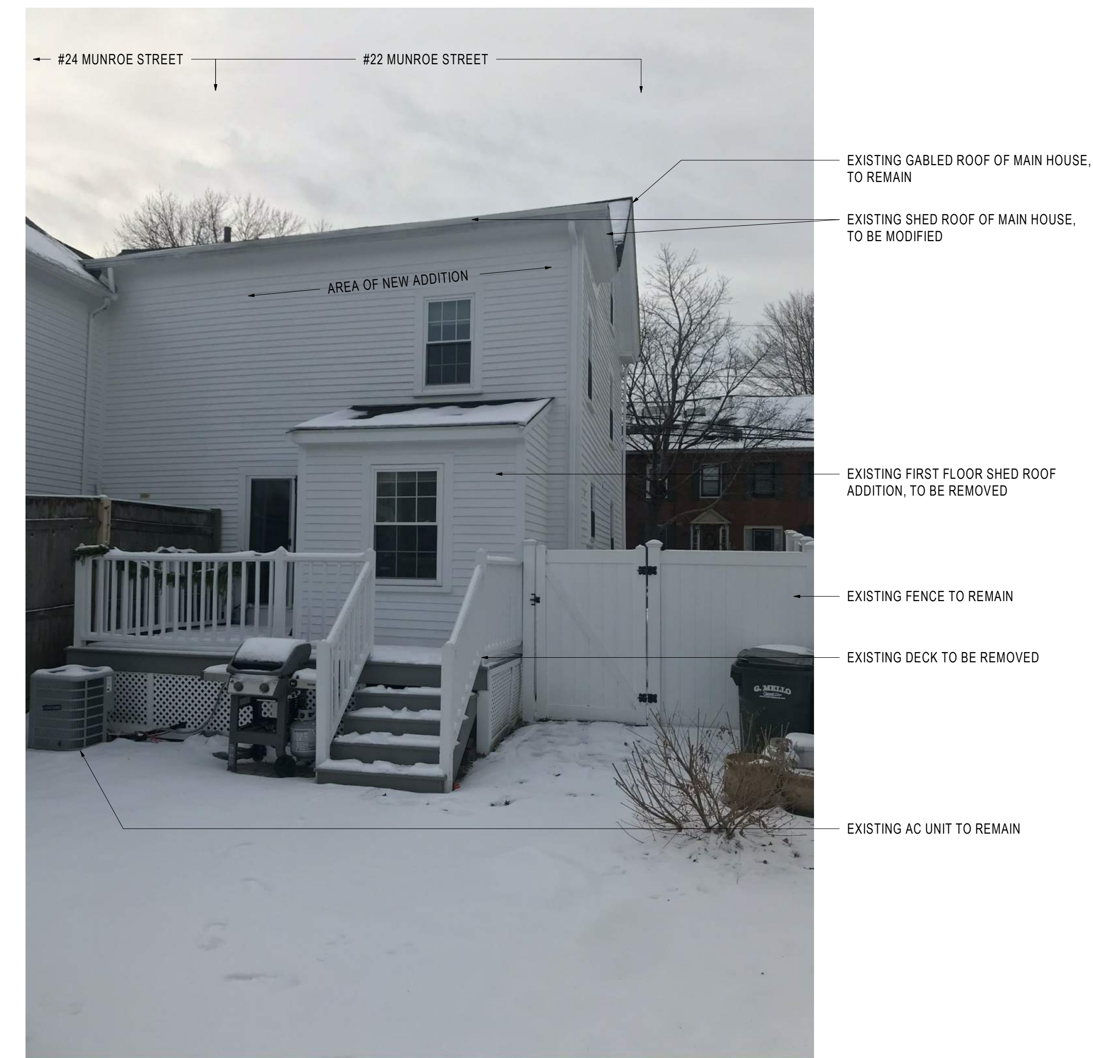
BACKYARD OF 22 MUNROE (NORTH FACADE)
