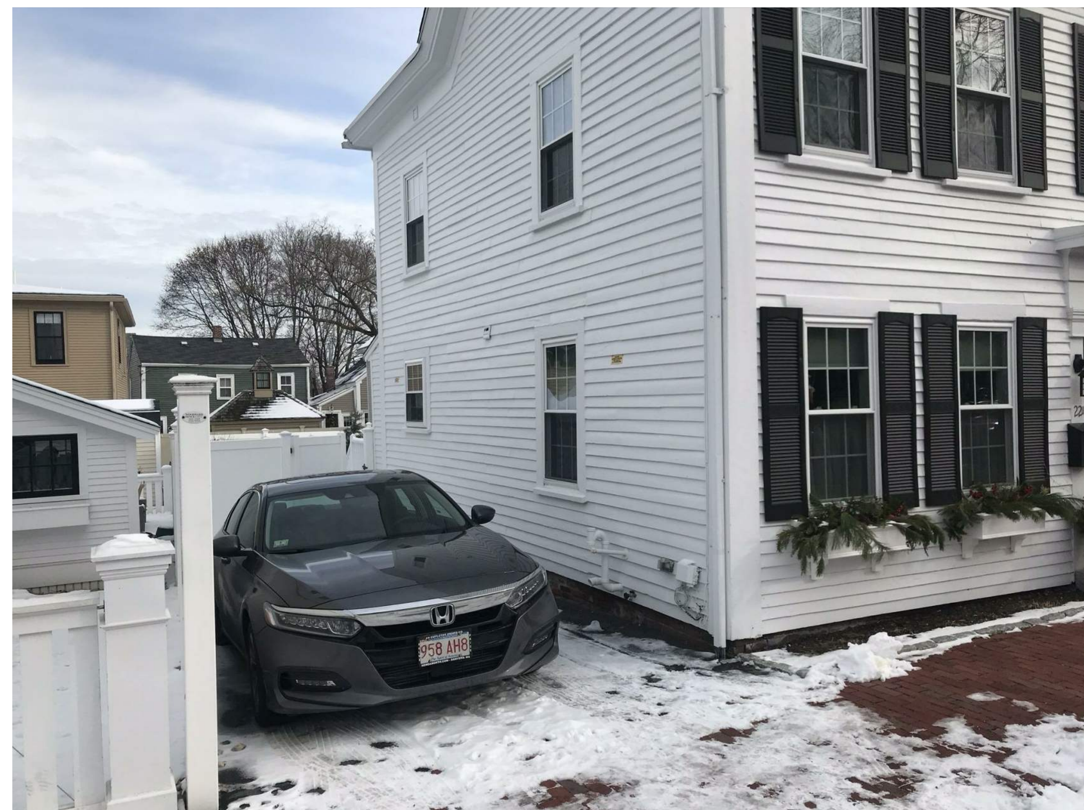
DRIVEWAY SIDE OF 22 MUNROE (WEST FACADE)
