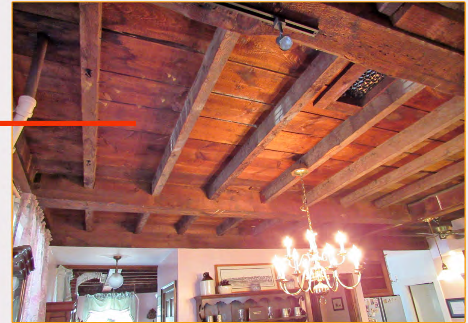
4. Existing Kitchen + Dining Ceiling
