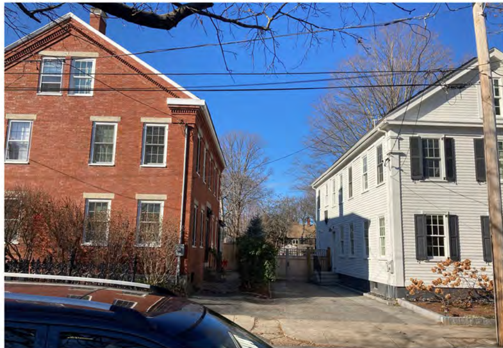
18-20 OLIVE STREET (LEFT); 16 OLIVE STREET (RIGHT). 15' APART.
