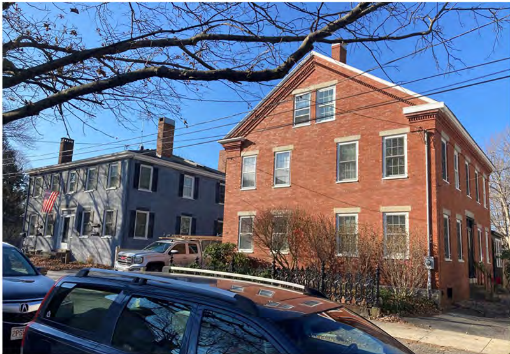
22-24 OLIVE STREET (LEFT); 18-20 OLIVE STREET (RIGHT). 25' APART.
