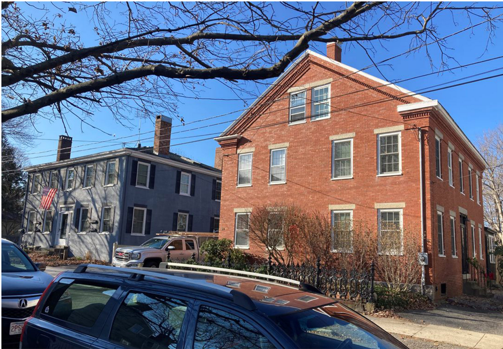
22-24 OLIVE STREET (LEFT); 18-20 OLIVE STREET (RIGHT). 25' APART.
