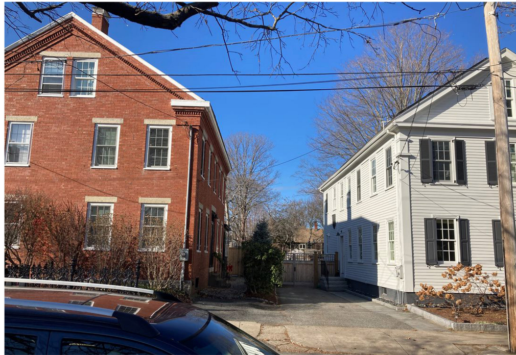
18-20 OLIVE STREET (LEFT); 16 OLIVE STREET (RIGHT). 15' APART.
