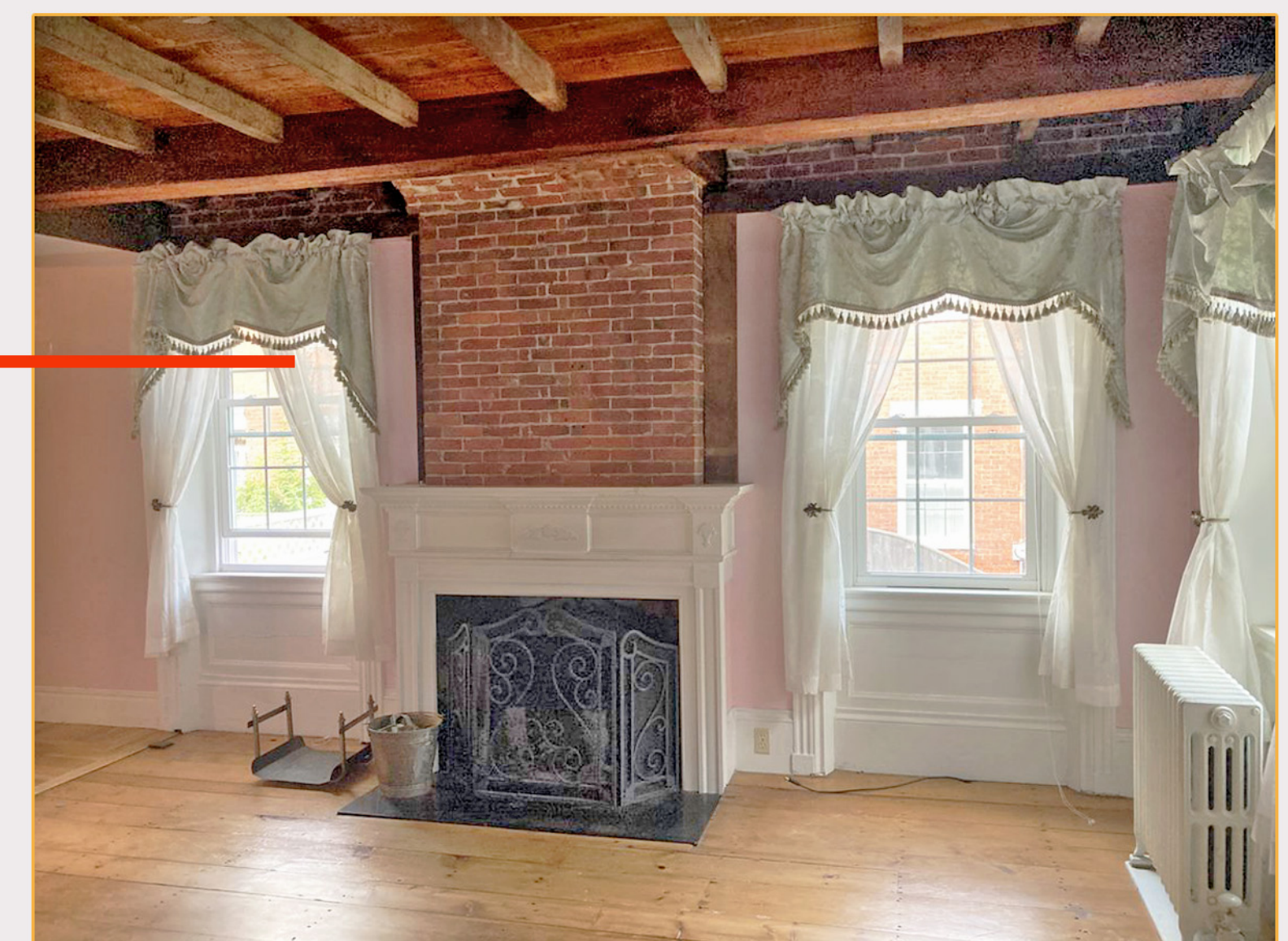
7. Existing Parlor/Study Fireplace, Windows, and Exposed Timber Ceiling
