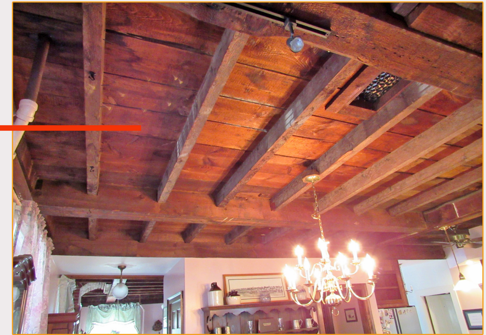
4. Existing Kitchen + Dining Ceiling
