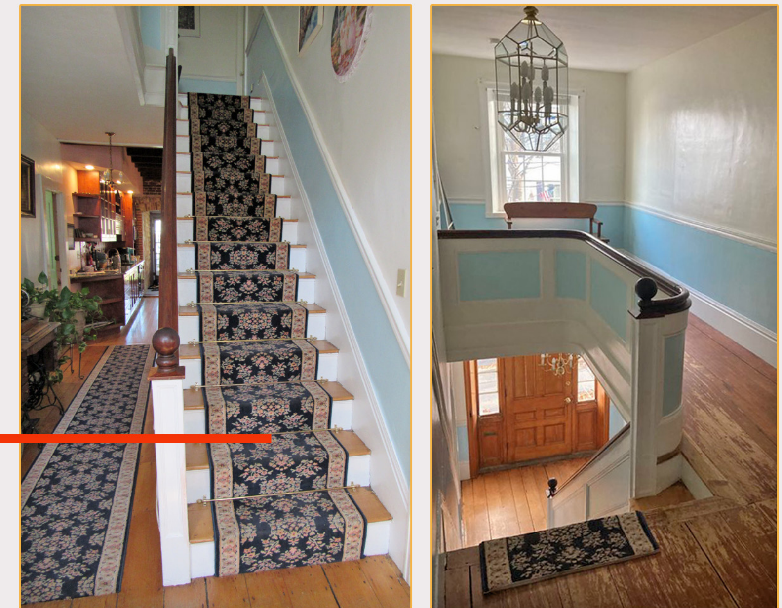
5+6. Existing Central Main Stair and Primary Hallway, Floors 1 + 2
