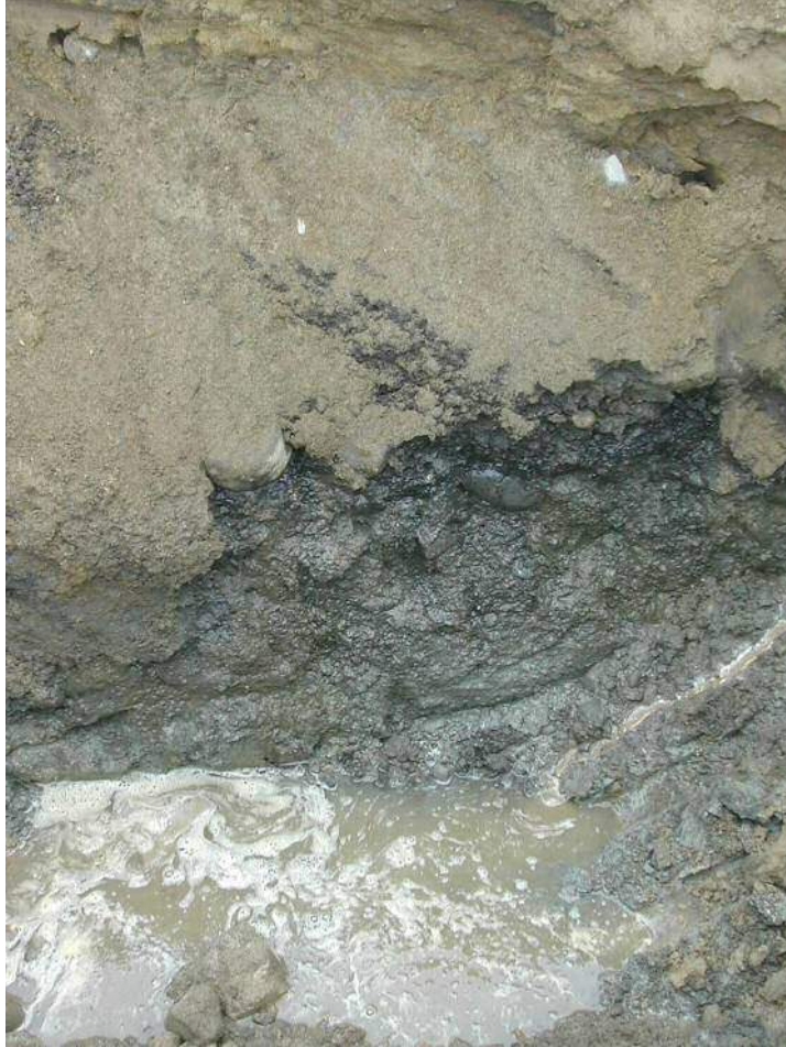
Photo 9: Bottom of TP-9 excavation.
