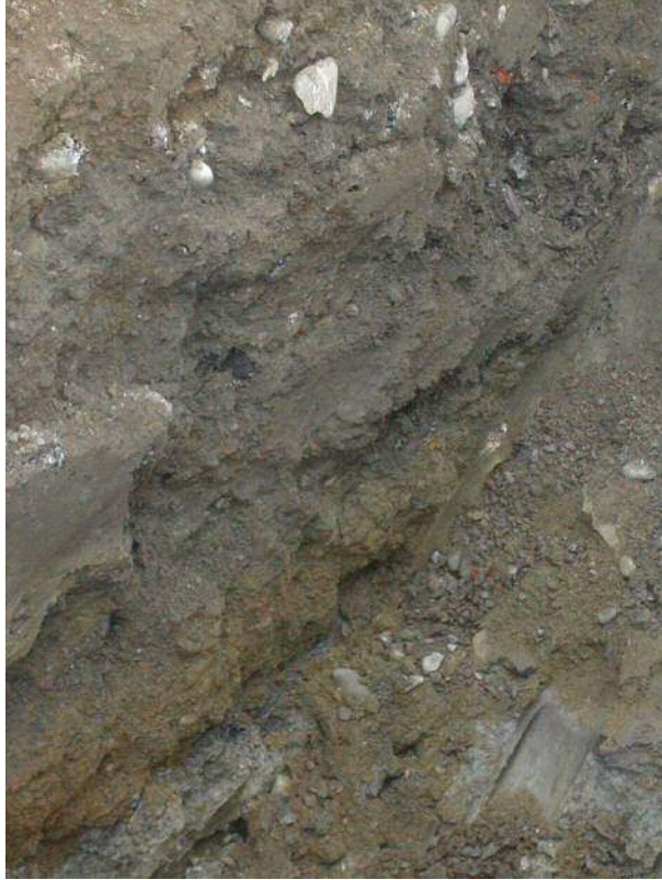
Photo 3: Eastern sidewall of Test Pit TP-5.
