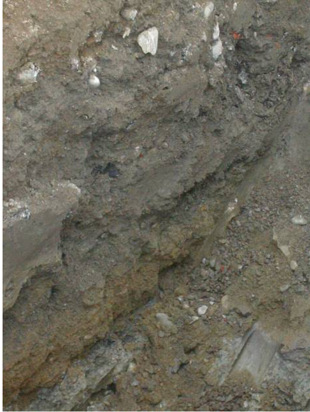
Photo 3: Eastern sidewall of Test Pit TP-5.
