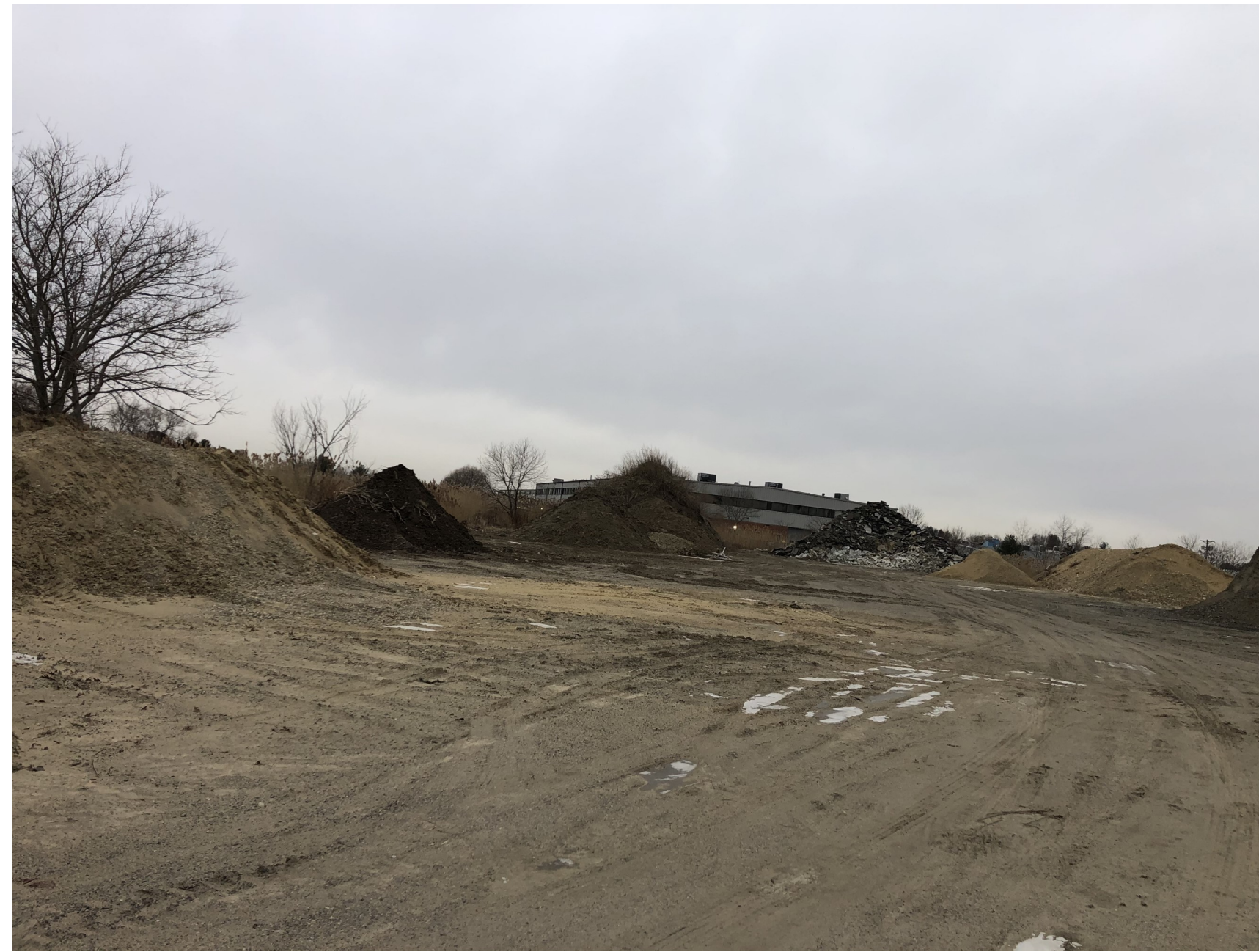
Looking into the site
