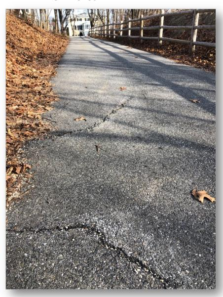
Several stretches of asphalt along the original Clipper City Rail Trail are in need of repair due to the effects of damage by tree roots. Locations needing replacement include the High Street spur going from High to the main trail pathway; north of the Low Street bridge by the granite steps; south of the Low Street bridge; near the locomotive sculpture; north of the bridge over Merrimack Street; south of the rail road bridge from the bridge to the granite steps at Strong Street.
