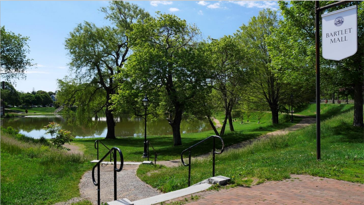
The current stairs and eroding walkway present accessibility barriers to lower levels of Bartlet Mall and will be replaced with an ADA compliant drive depicted below.
