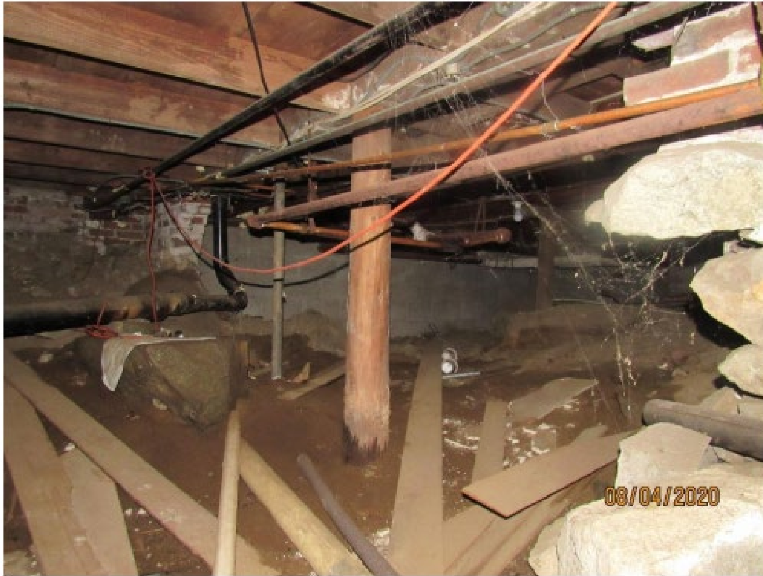
Photo 7 Antiquated timber framing with posts extending below grade and foundation walls demolished
