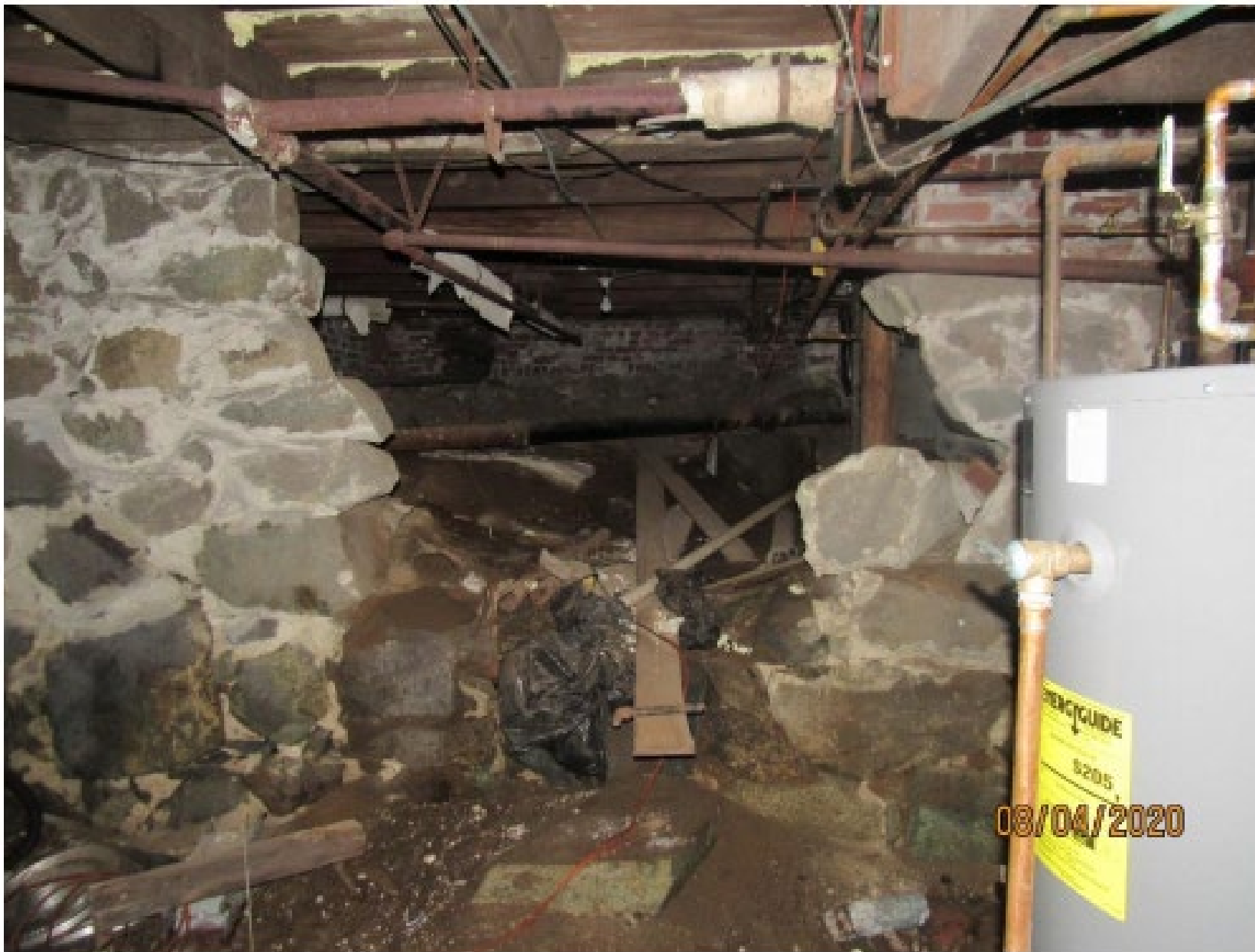
Photo 8 Foundation walls partially demolished to allow additions
