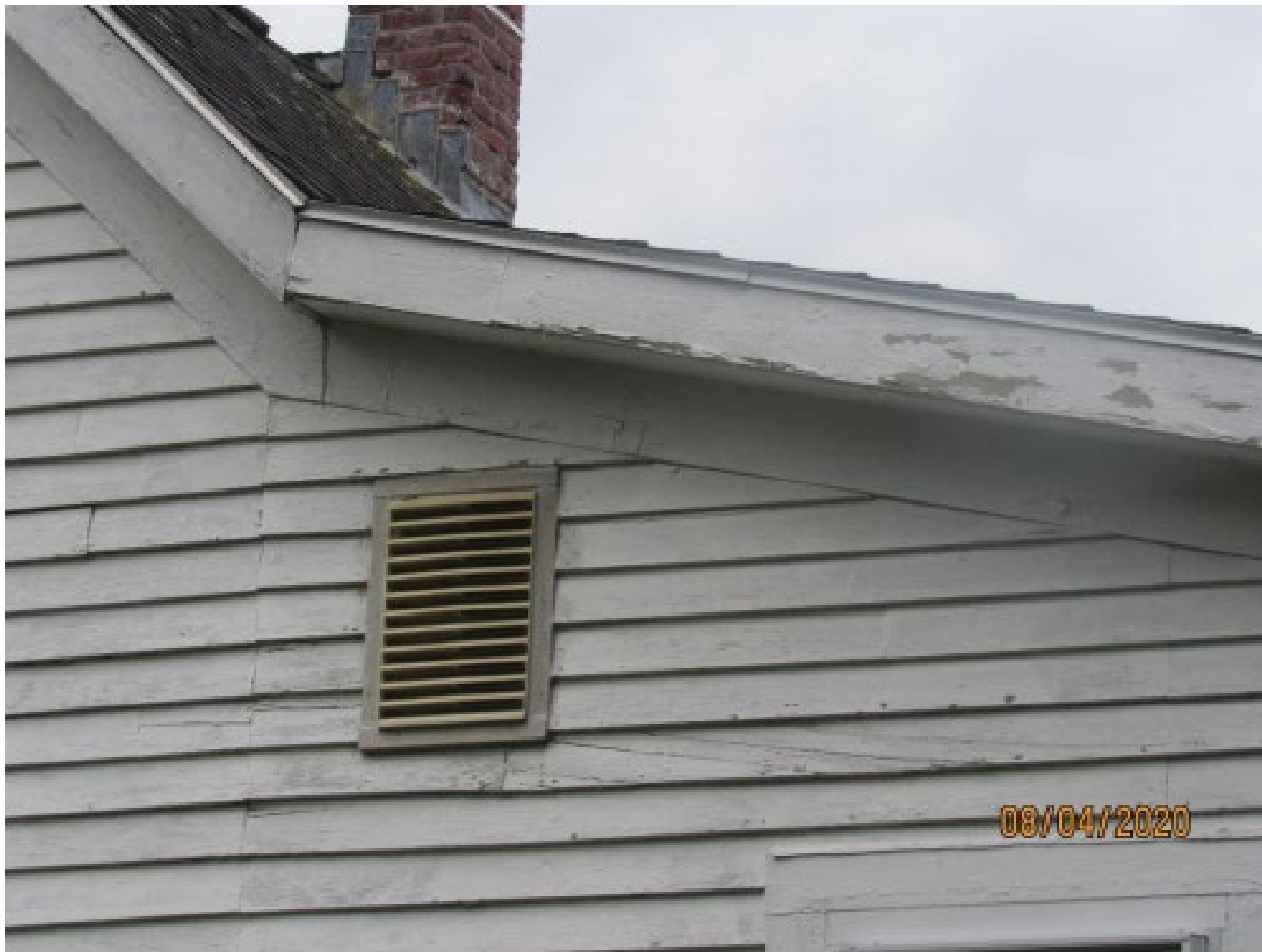
Photo 11 Ventilation beneath the roof
