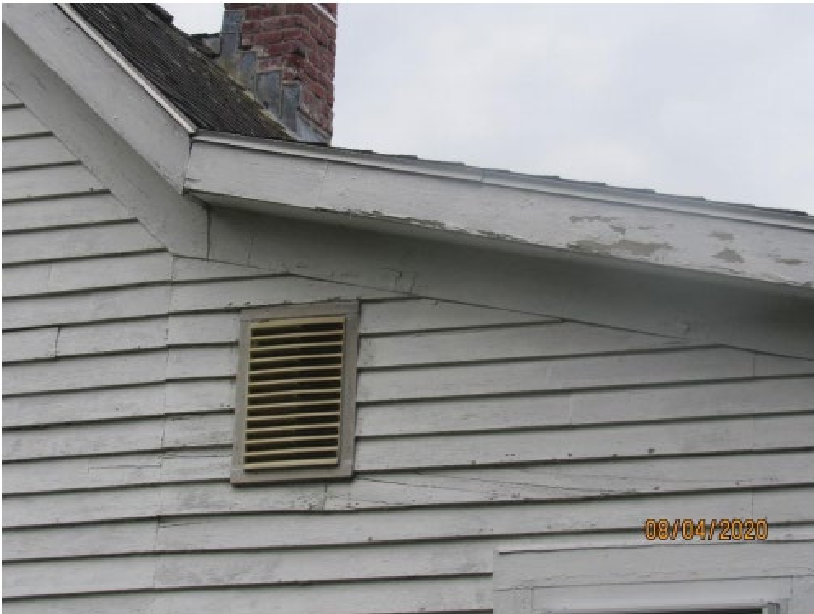
Photo 11 Ventilation beneath the roof
