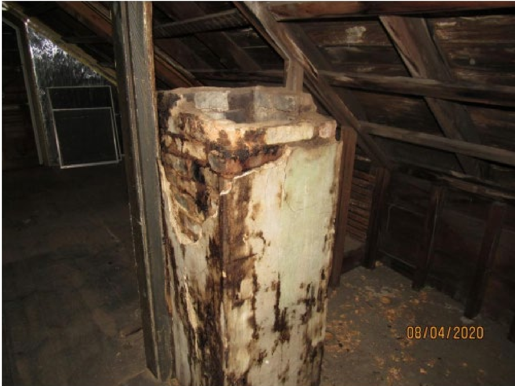
Photo 9 Balloon framed walls to support roof and chimney demolished and abandoned in the attic
