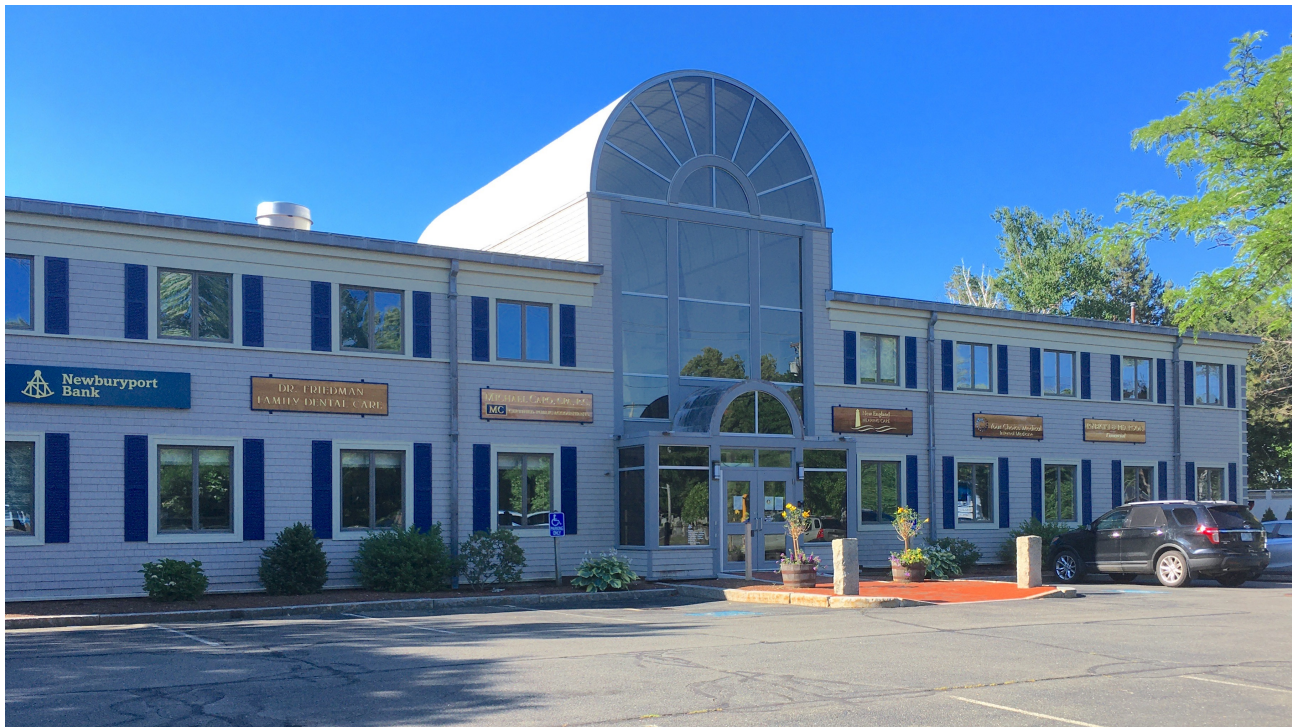
Illustration 1: A commercial building on Storey Ave.
