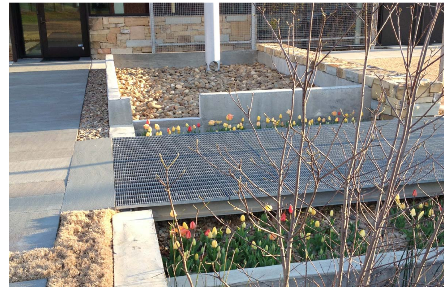
6 STORM WATER RETENTION WALL - CHARACTER NTS
