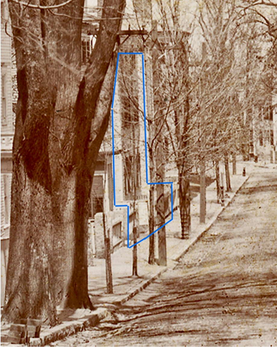
Figure 1a, detail of figure 1, showing fencing in front of the walkway between 16 and 14 Fruit Street as well as in front of each building
