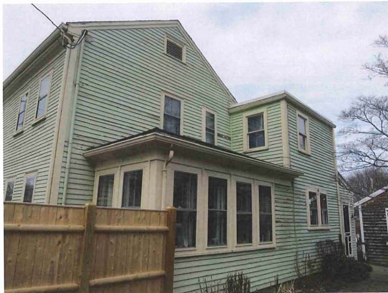
17_View north showing southeast elevation from west end
