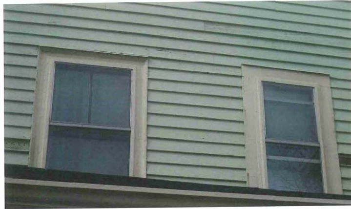
20_View northwest showing southeast elevation - detail of second floor windows
