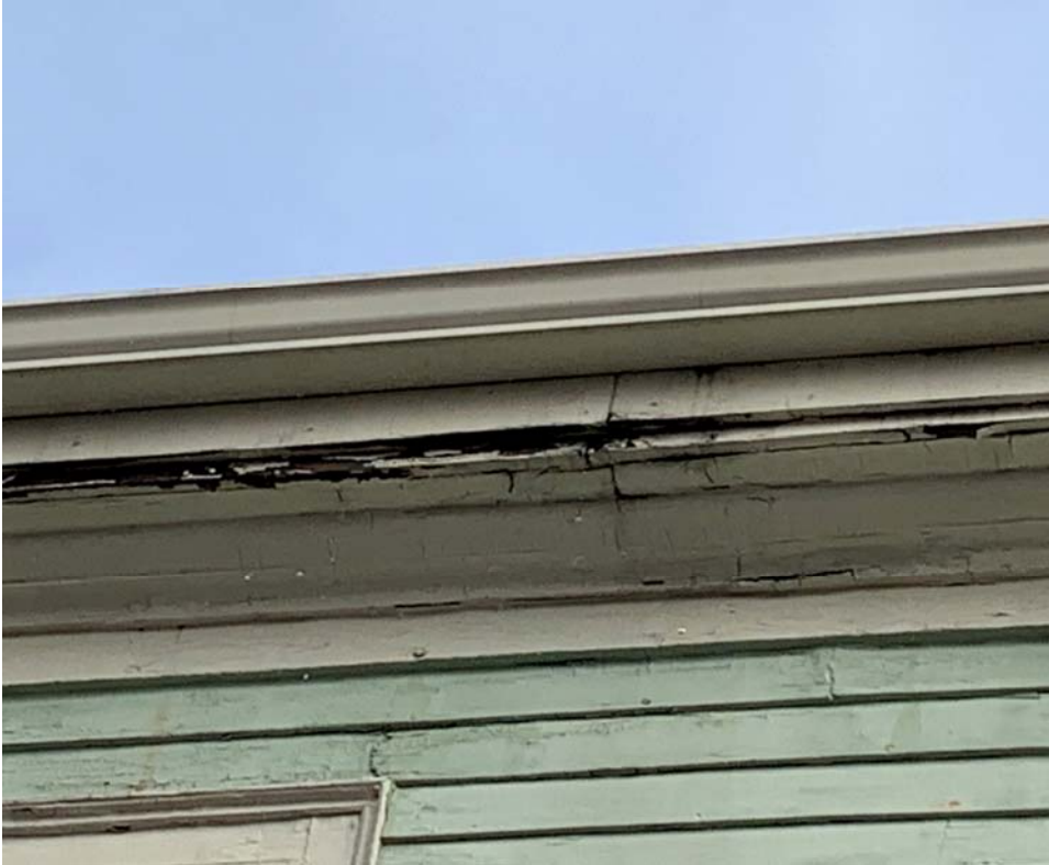
Figure 8A – Soffit and Trim Repair
