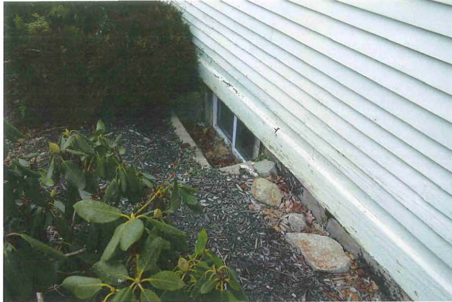
12_View northeast showing principal facade (northwest elevation) - detail of foundation and basement window at north end
