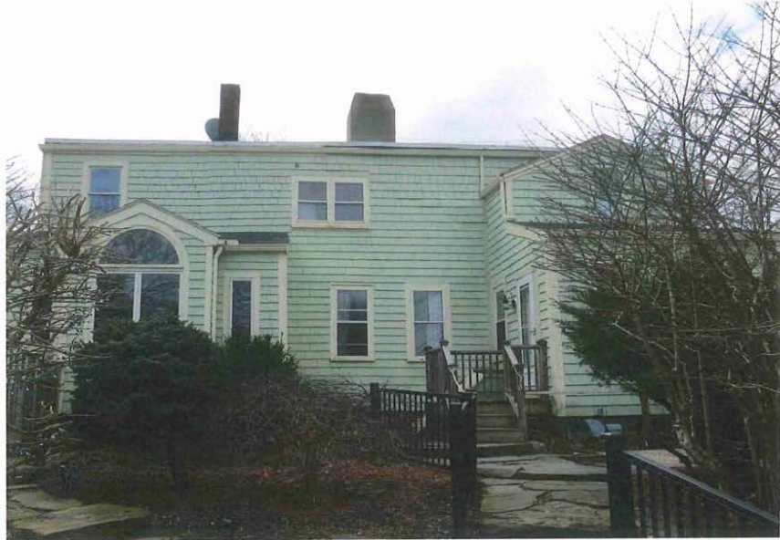
22_View southwest showing rear (southeast) elevation
