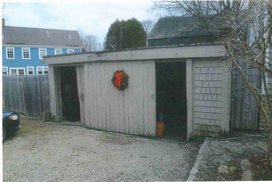
30_View southeast showing northwest elevation of shed
