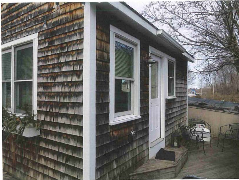
29_View northeast showing southeast elevation of non-historic guesthouse
