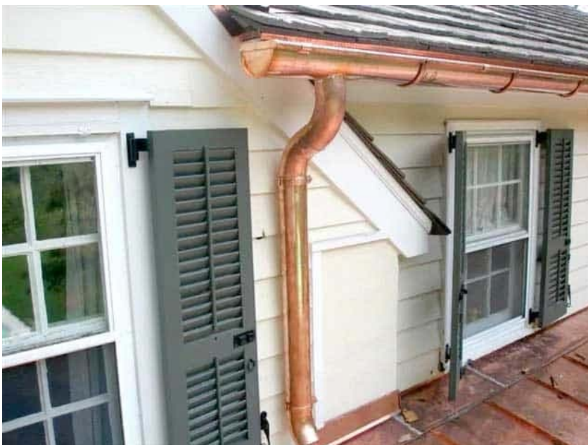
Figure 7 – Examples of Gutters and Downspouts
