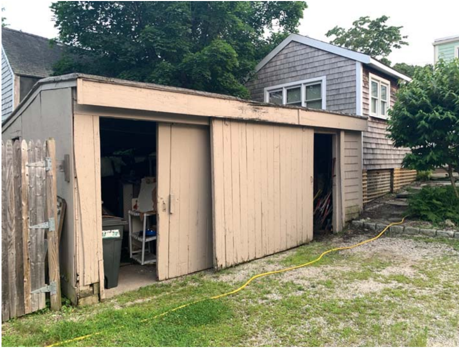
Figure 10 – Rear Shed to be Removed
