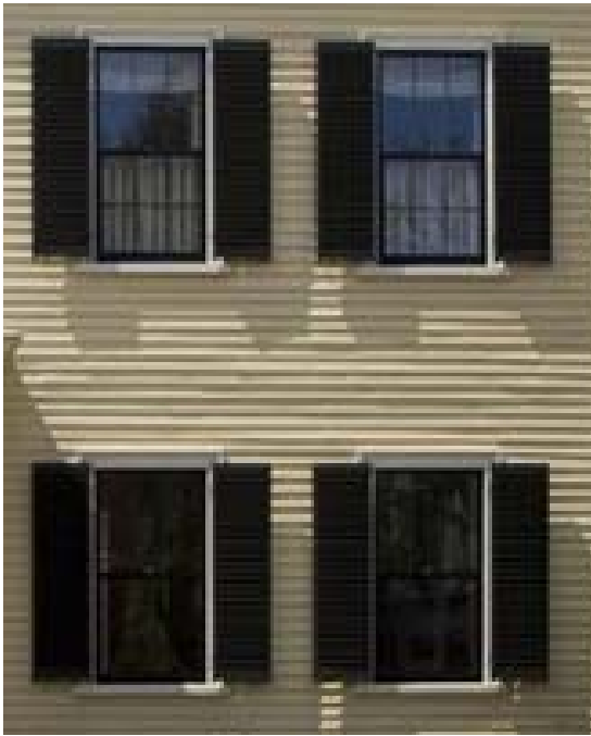
Figure 6 – Example of Federal-Style Shutters
