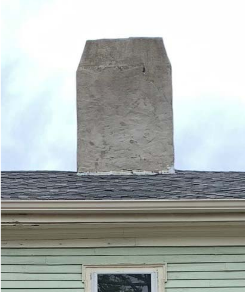
Figure 4 – Chimney Repair and Full Preservation (including the Interior)
