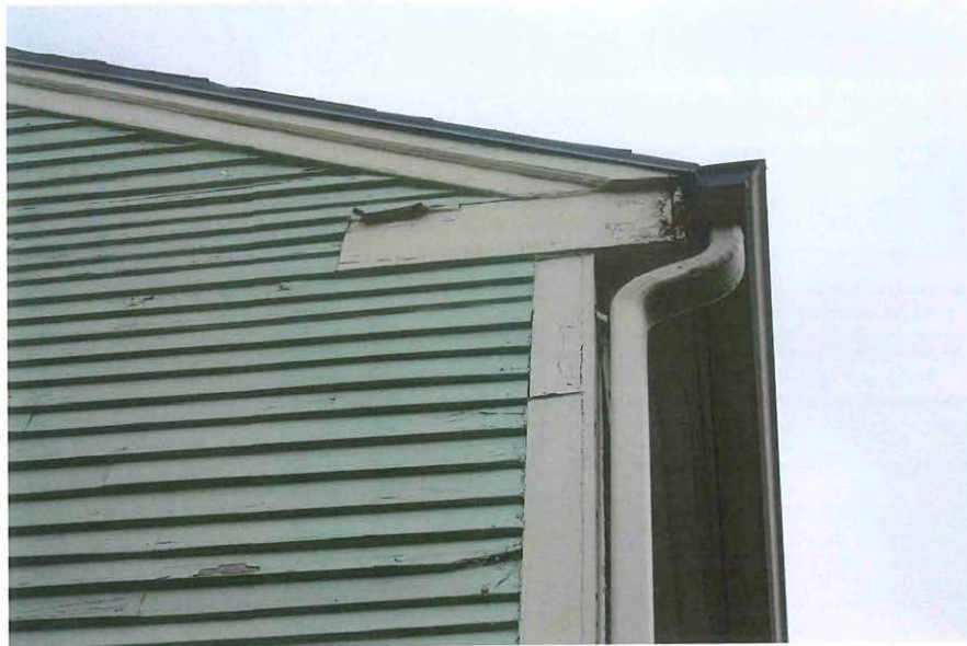
14_View southeast showing northwest elevation - detail of corner board, fascia, and return at gable
