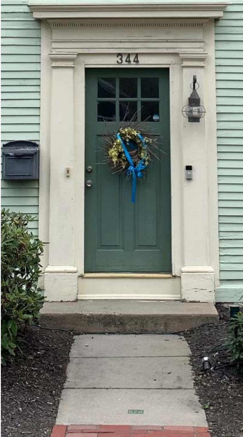
Figure 5 – Walkway Preservation and Step Replacement
