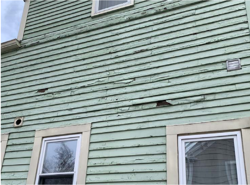
Figure 8B – Clapboard Repair
