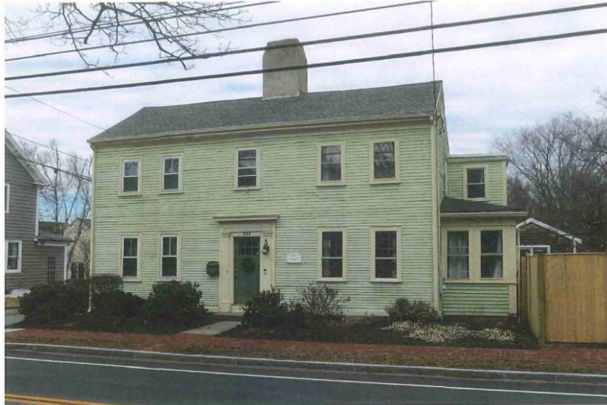
5_View northeast showing principal facade (southwest elevation)
