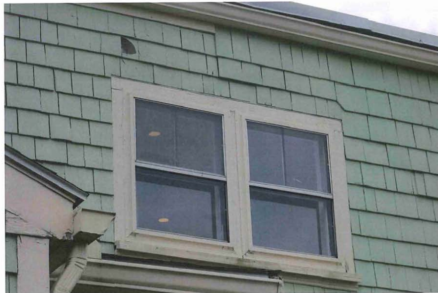
25_View southwest showing rear (southeast) elevation - detail of central bays at second floor
