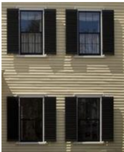
Figure 6 – Example of Federal-Style Shutters
