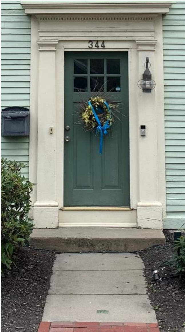
Figure 5 – Walkway Preservation and Step Replacement
