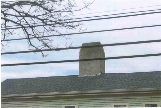
7_ View northeast showing chimney on main block and asphalt roof
