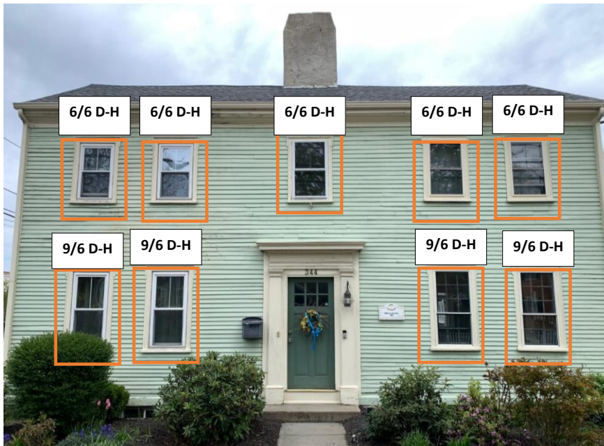
Figure 1A - Window Replacement on the Merrimac Street Facade
