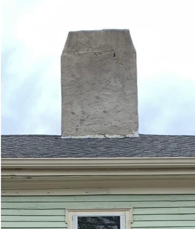
Figure 4 – Chimney Repair and Full Preservation (including the Interior)
