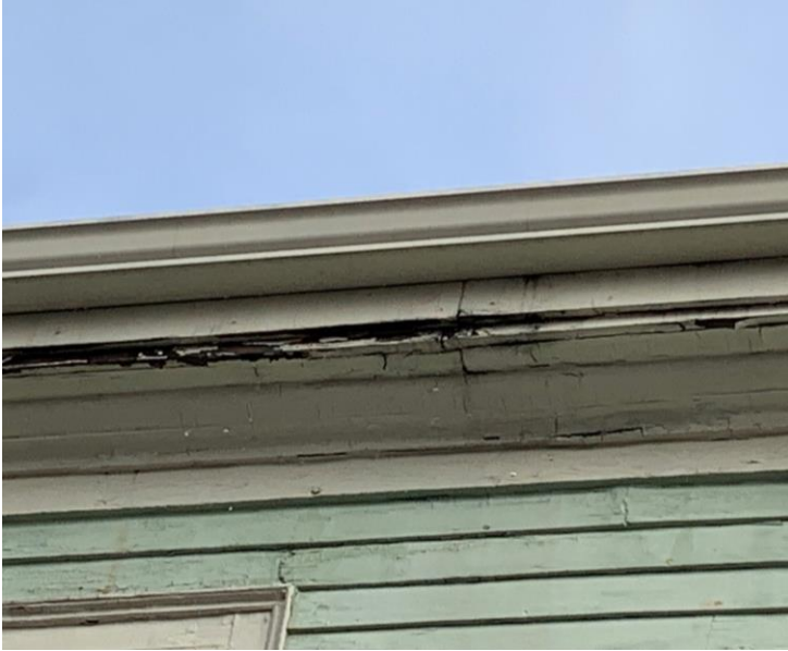
Figure 8A – Soffit and Trim Repair
