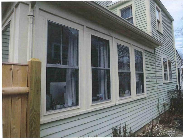
19_View north showing southeast elevation - detail of enclosed porch
