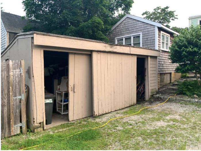
Figure 10 – Rear Shed to be Removed
