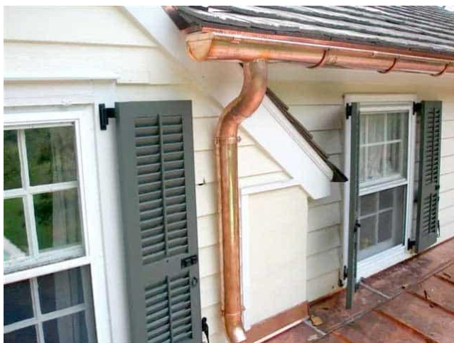
Figure 7 – Examples of Gutters and Downspouts
