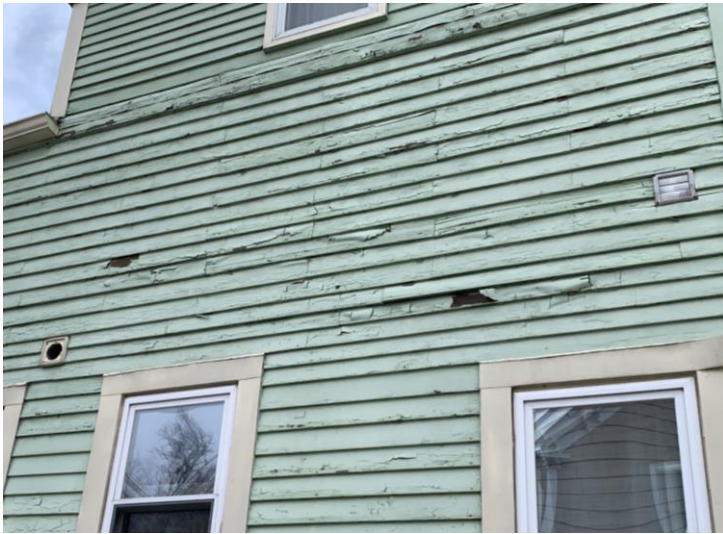
Figure 8B – Clapboard Repair
