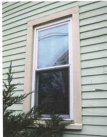
15_View southeast showing northwest elevation - detail of typical window
