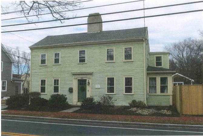
5_View northeast showing principal facade (southwest elevation)
