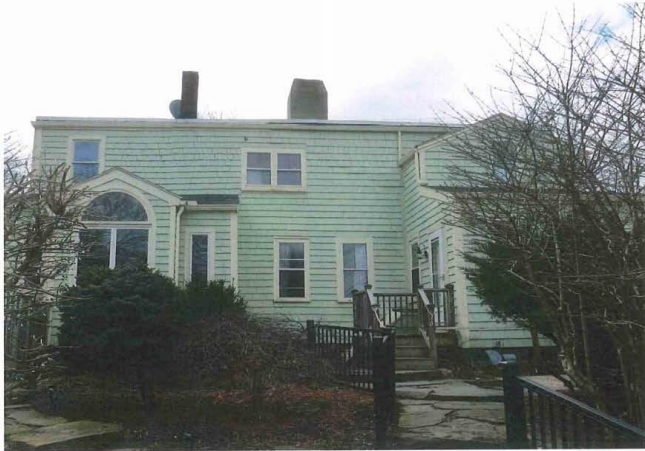
22_View southwest showing rear (southeast) elevation
