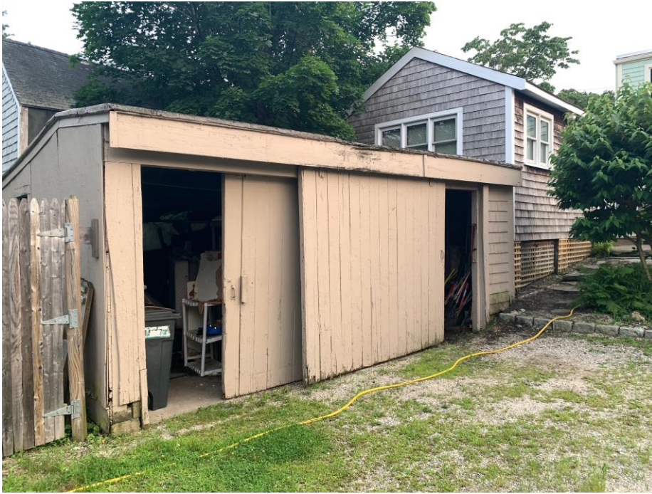
Figure 10 – Rear Shed to be Removed
