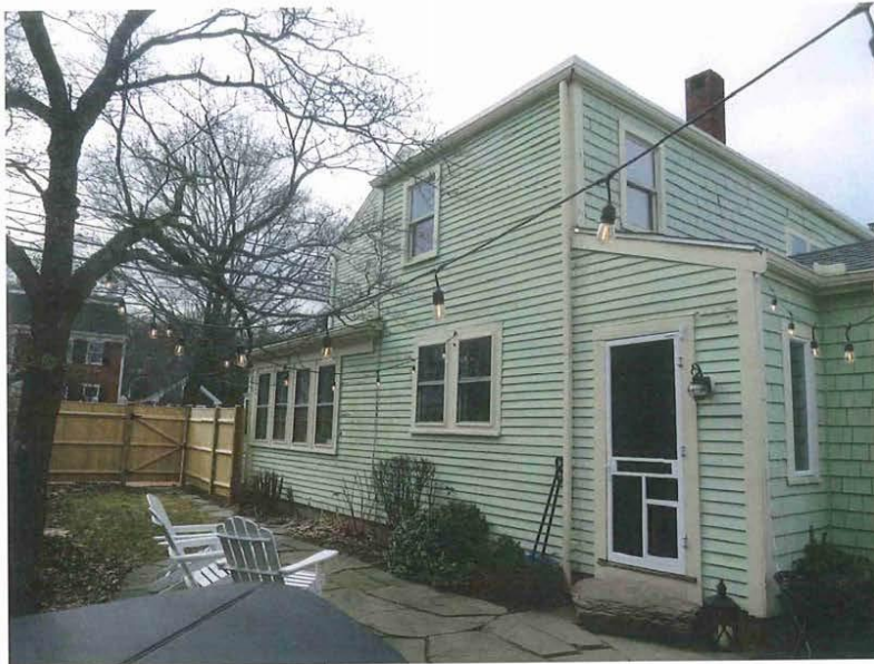
18_View northwest showing southeast elevation from east end
