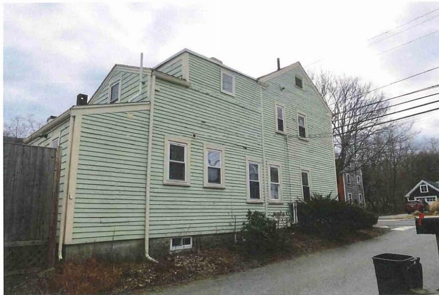
13_View southwest showing northwest elevation
