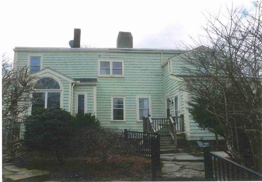
22_View southwest showing rear (southeast) elevation
