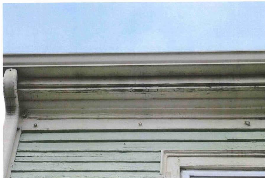
8_ View northeast showing principal facade (northwest elevation) - detail of cornice
