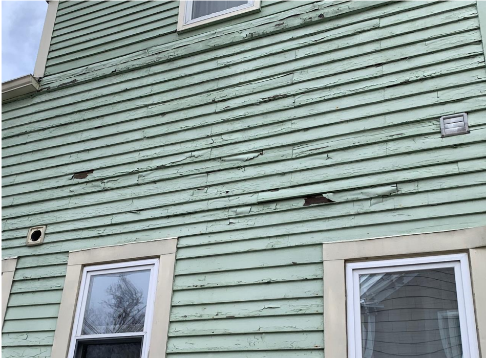
Figure 8B – Clapboard Repair
