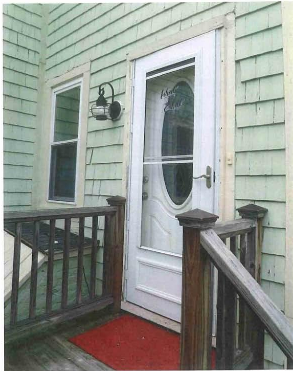
26_ View northwest showing southeast face of rear ell/ northeast addition - detail of porch, entry, and window
