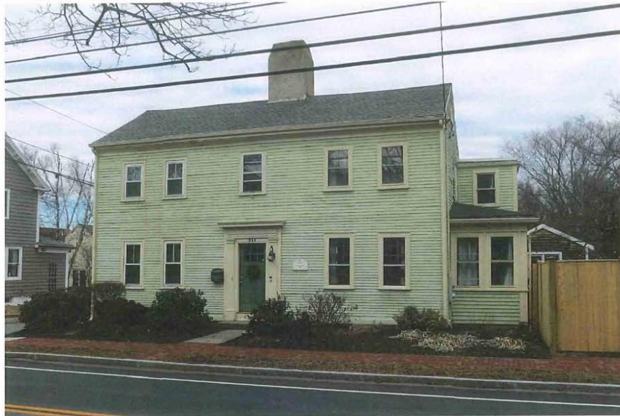
5_View northeast showing principal facade (southwest elevation)
