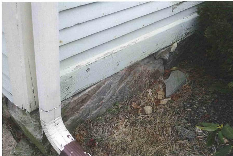
6_View northeast showing principal facade (southwest elevation) - detail of foundation
