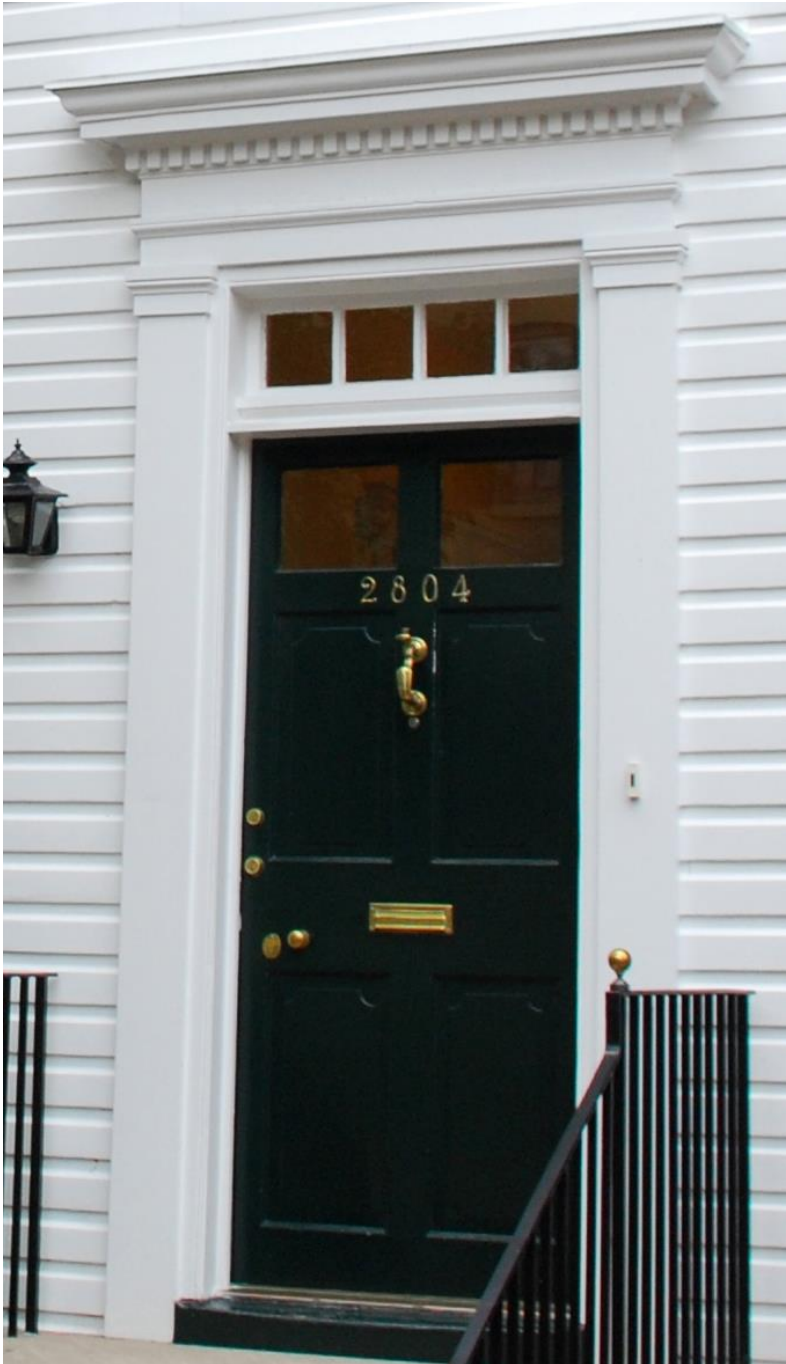
Figure 3 – Example Federal-Style Door Replacement
