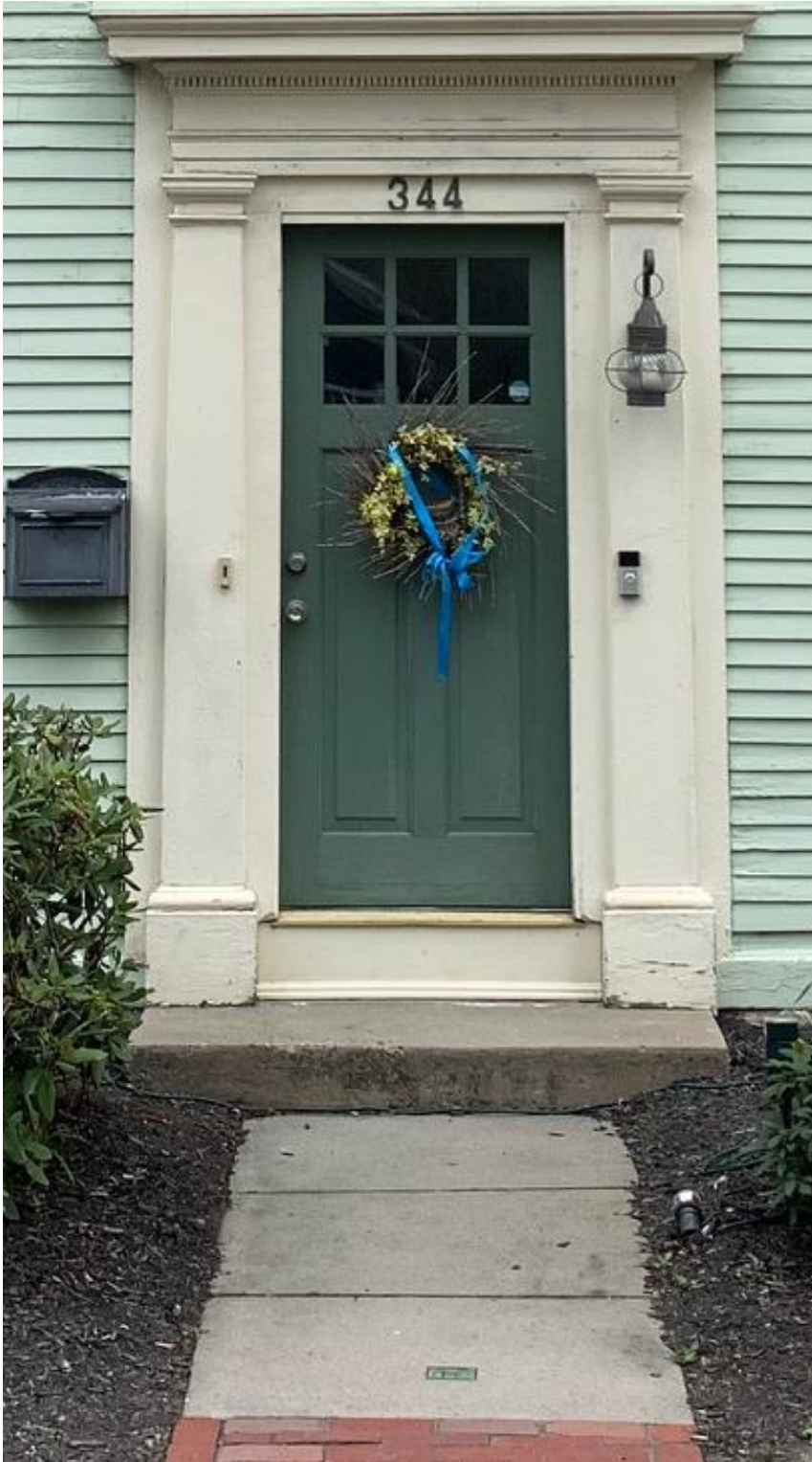
Figure 5 – Walkway Preservation and Step Replacement
