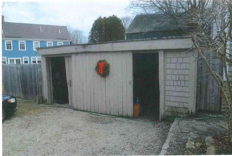
30_View southeast showing northwest elevation of shed
