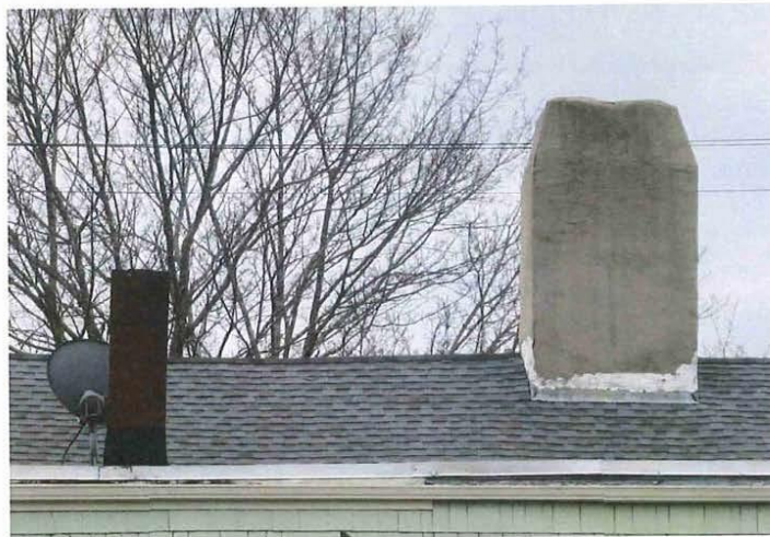
27_ View northwest showing chimneys on roofs of main block (right) and rear addition (left)
