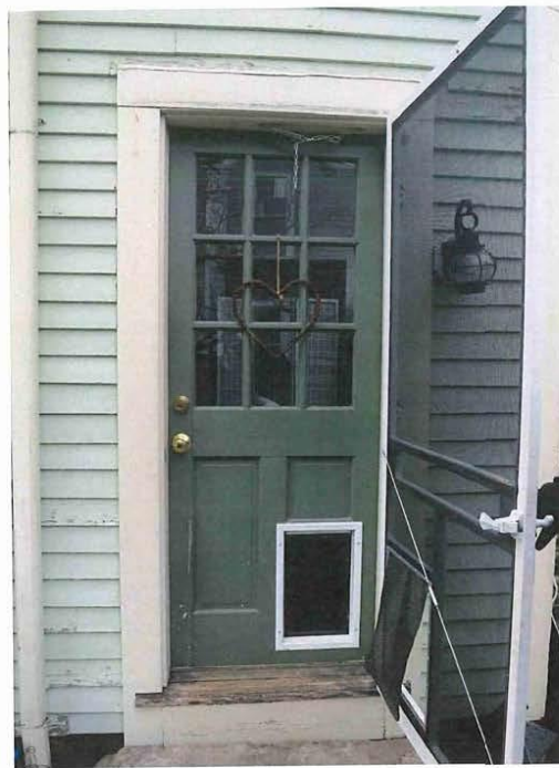
21_View northwest showing southeast elevation - detail of entry at east end
