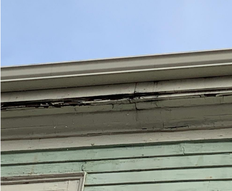
Figure 8A – Soffit and Trim Repair
