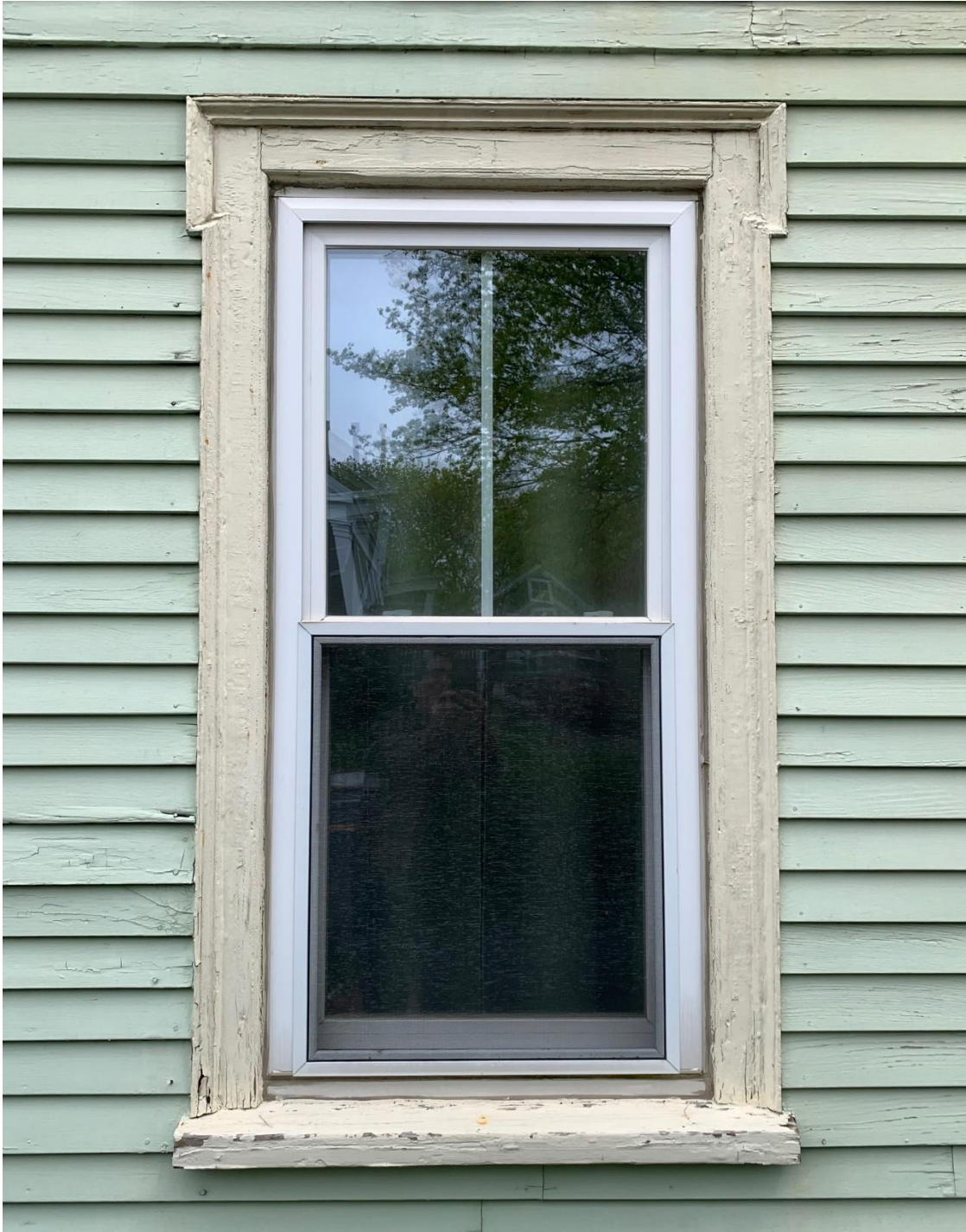
Figure 2 – Existing Window Casing on the Merrimac Street Facade
