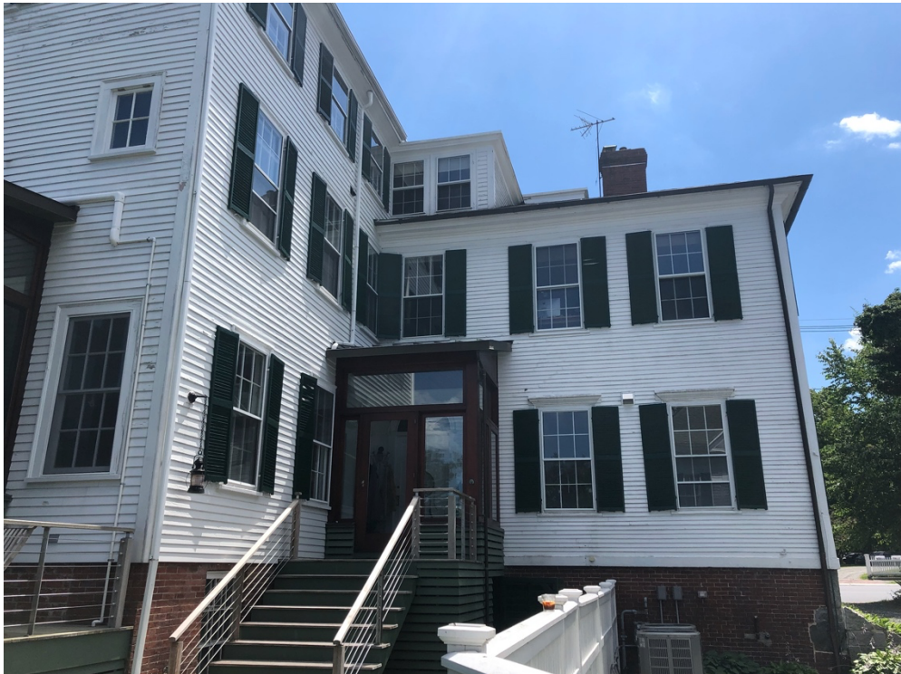
Photo 6, Main House, North Elevation, July 2019
