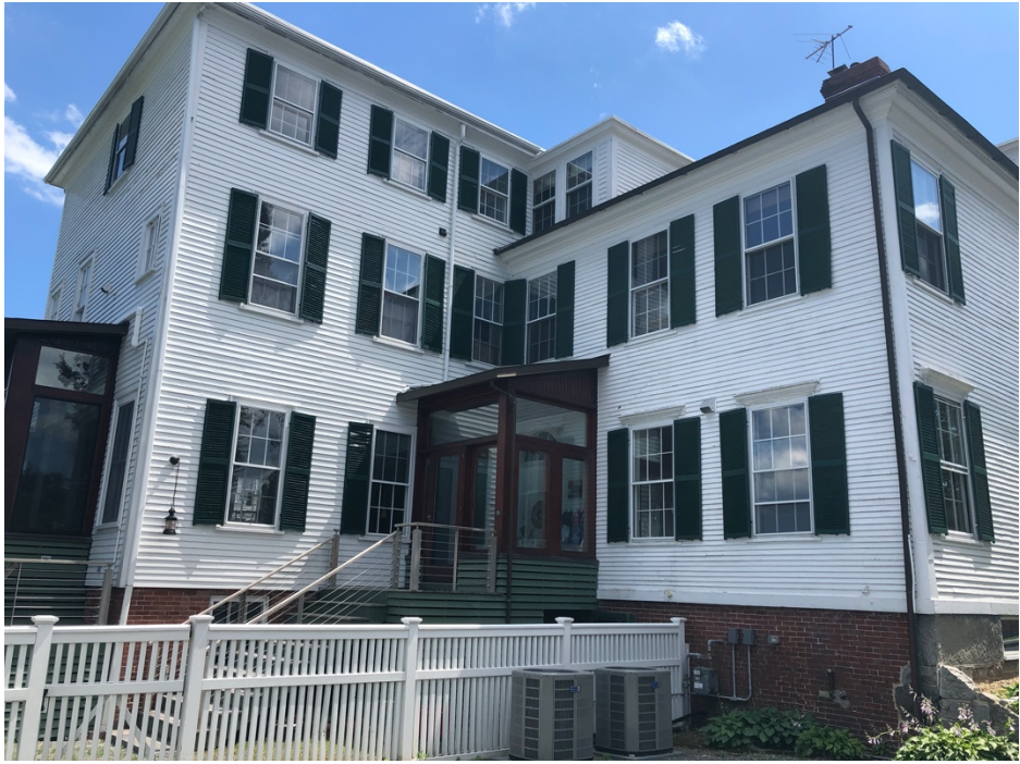
Photo 7, Main House, South West Elevation, July 2019
