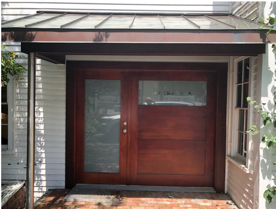
Photo 9, Carriage House, South Elevation detail, July 2019
