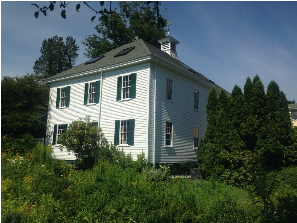
Photo 12, Carriage House, North East Corner, July 2019
