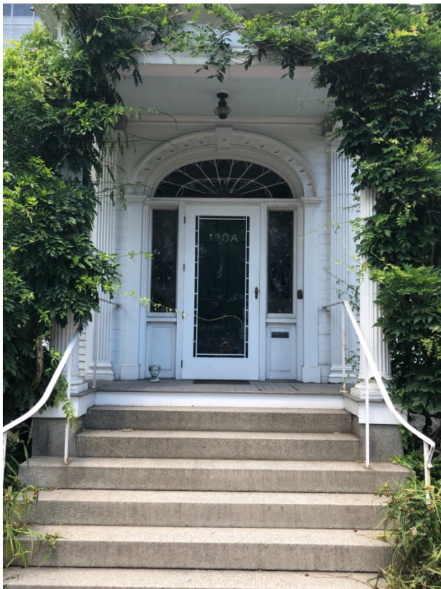
Photo 2, Main House, South Elevation, July 2019
