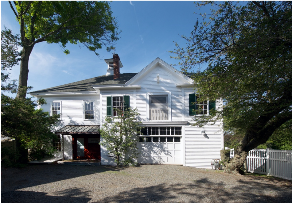
Photo 8, Carriage House, South Elevation, July 2019
