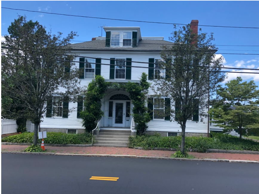
Photo 1, Main House, South Elevation, July 2019
