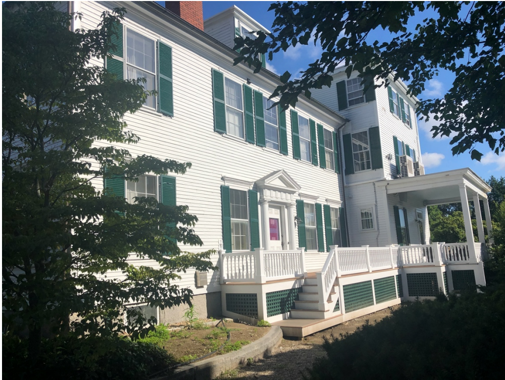
Photo 3, Main House, East Elevation, July 2020
