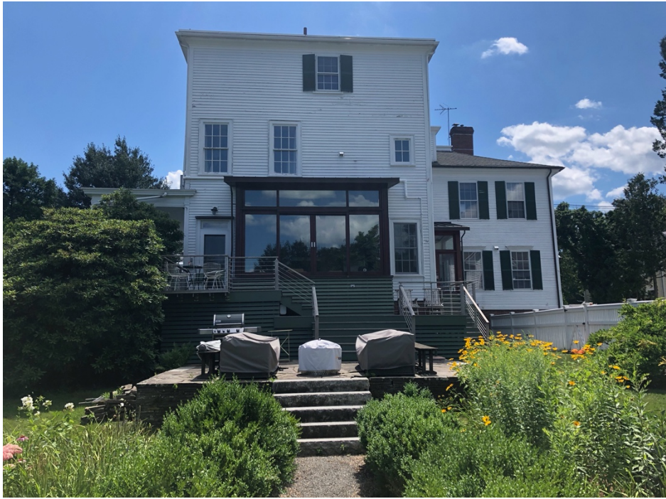
Photo 7, Main House, South Elevation, July 2019
