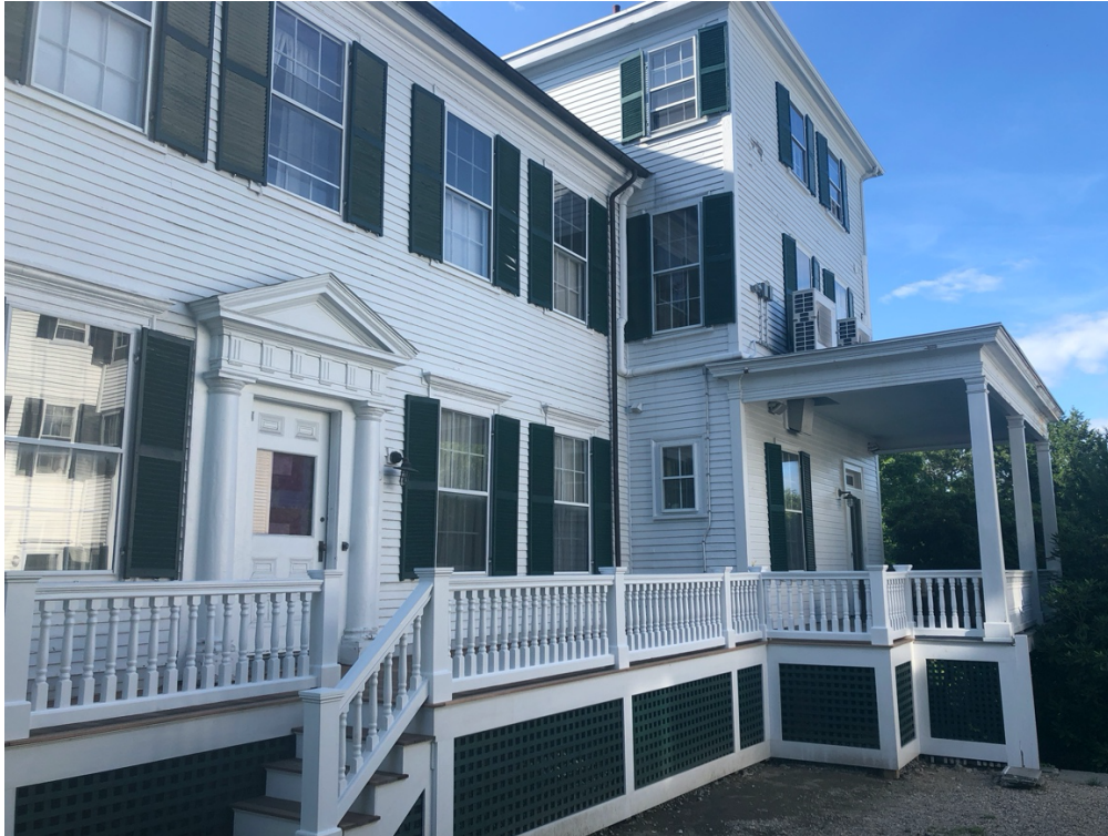
Photo 4, Main House, East Elevation, July 2020
