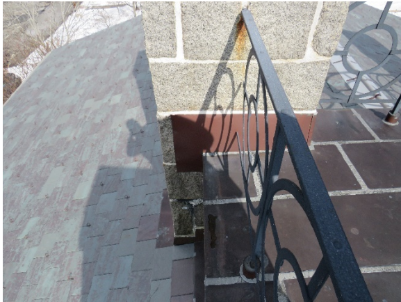
10. Observatory guardrail pitch pocket
