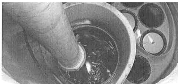
Vacuuming Sump Through MAW
