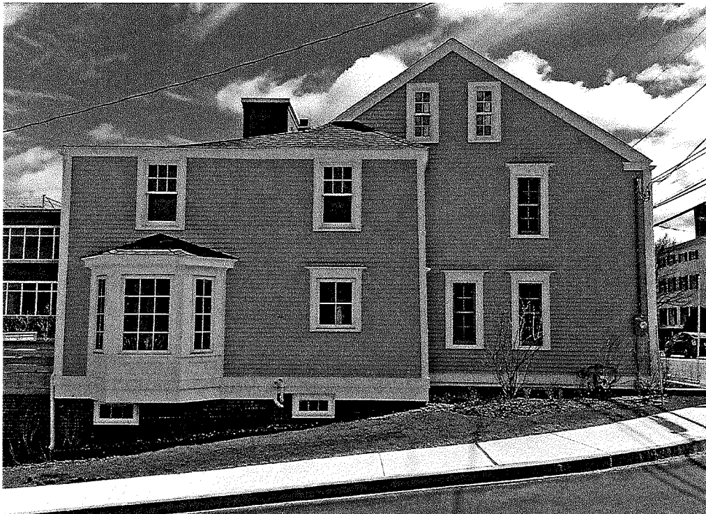
17. Left (north) elevation – April 2017
