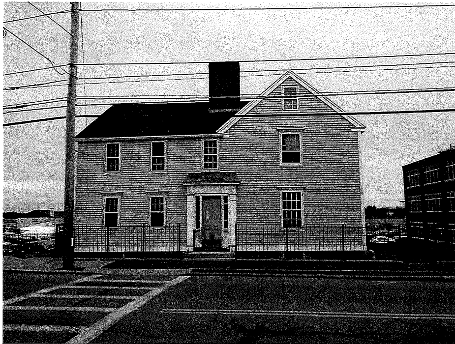
3. Street (west) elevation – April 2015
