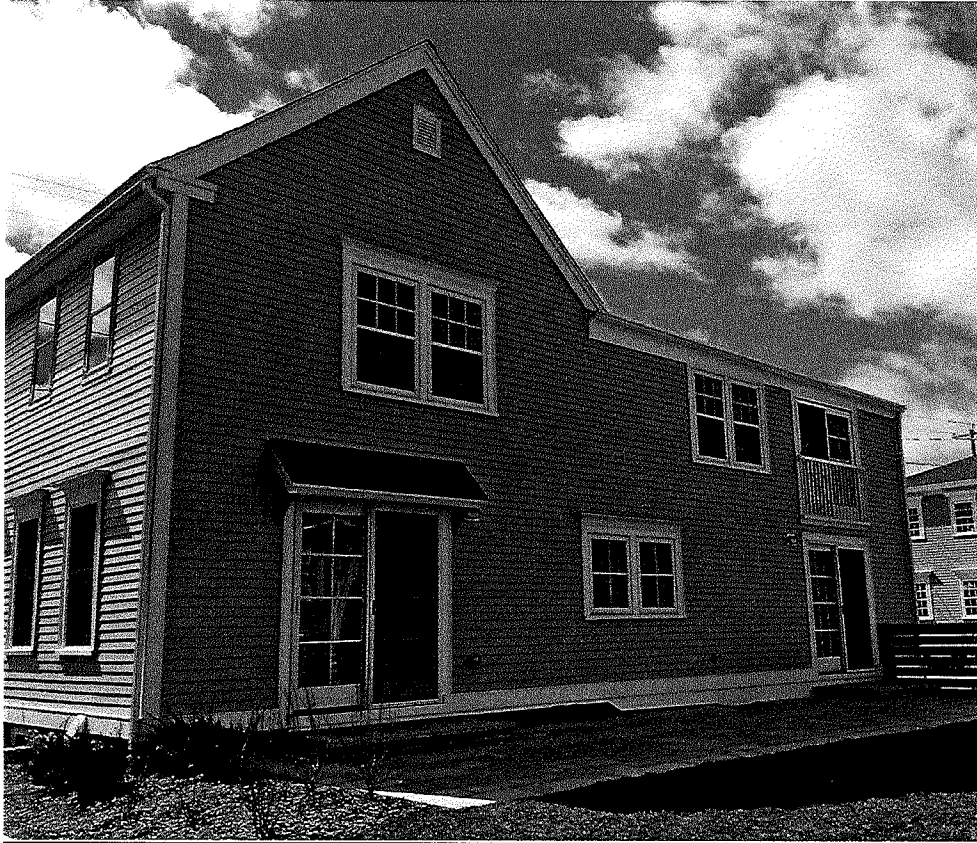
18. Rear (east) elevation – April 2017
