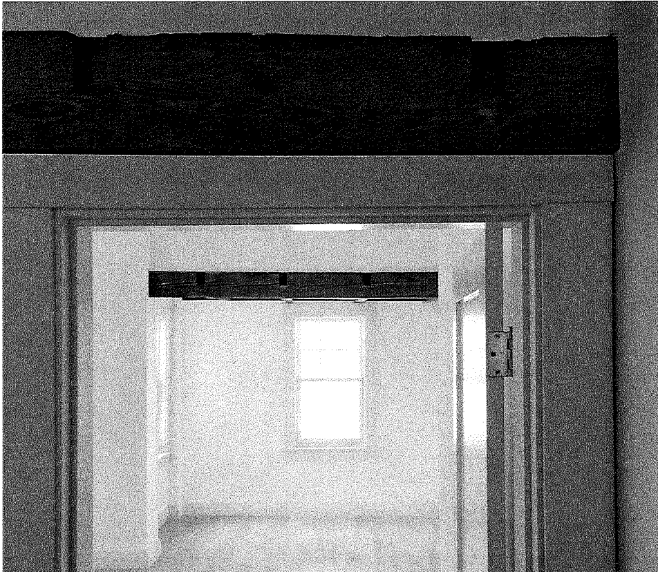
14. Exposed beams at second floor master bedroom – March 2017
