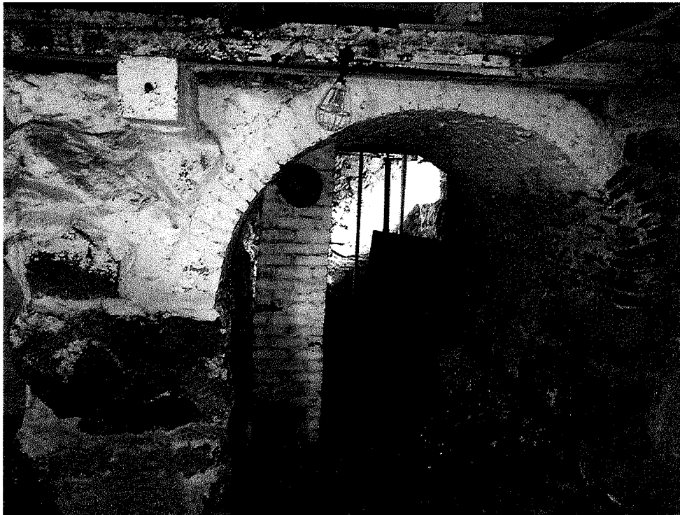
9. Basement arch and foundation – June 2015
