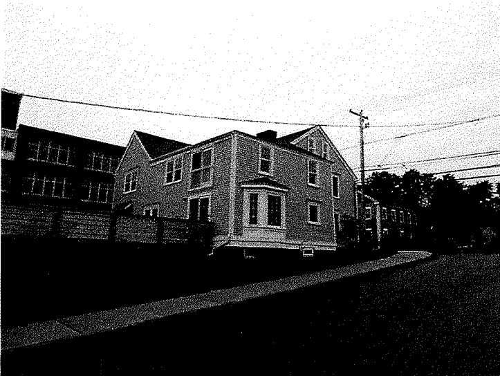
262-264 Merrimac Street, camera facing southwest
