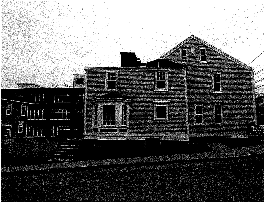
4. Left (north) elevation – April 2015
