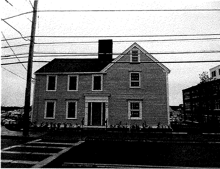
262-264 Merrimac Street, camera facing northeast
