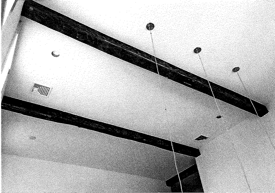
13. Exposed second floor beams – March 2017
