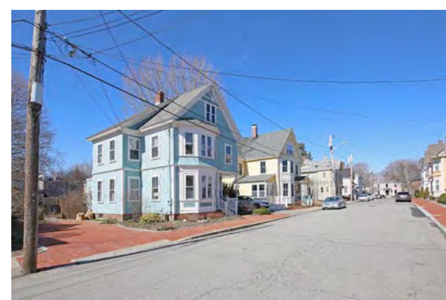
STREET VIEW: NORTHEAST CORNER
