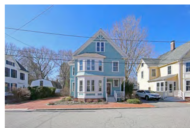
STREET VIEW: NORTH FACADE
