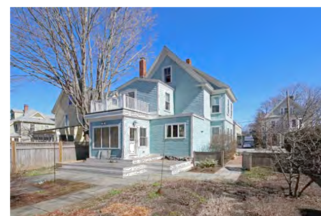
REAR VIEW: SOUTHEAST CORNER
