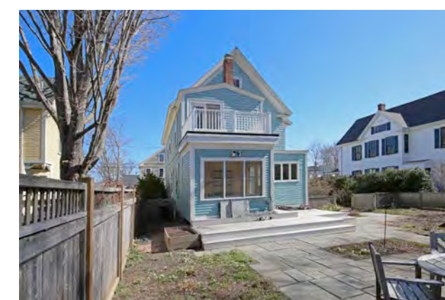
REAR VIEW: SOUTHWEST CORNER
