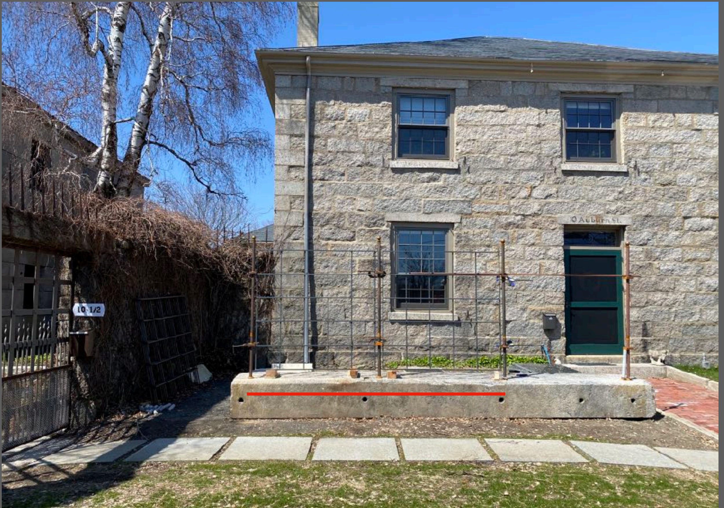
VIEW OF TWO PANELS FROM LAWN PANELS OF 1/2" STEEL ARE ABOVE RED LINE
