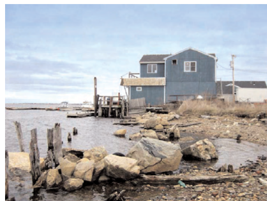
Collapsed seawall
