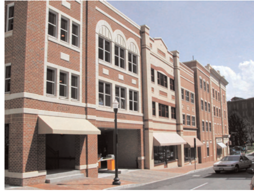
Parking garage with ground floor retail
