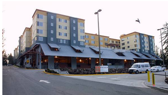
The Village at Overlake Station, a transit-oriented development in Redmond, Washington, includes two levels of covered parking with 536 parking stalls and 308 rental housing units affordable to households earning 60 percent of the area's median income. The garage provides shared parking for use by both residents and park-and-ride users. The site continues to operate as a park-and-ride lot and a major transit facility in the King County Metro Transit system.
