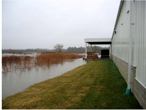
The Little River flooding at Bixby International, April 2004 (photo: Bob McLellan, Bixby International).
