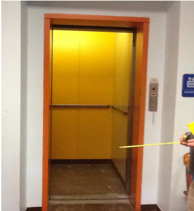
ELEVATOR WITH 32” DOOR OPENING
