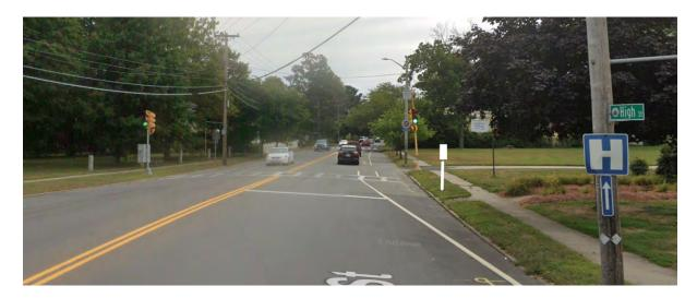
2. A Reduced Speed Limit Ahead sign west of the Three Roads intersection may be justified because vehicles rounding the wide curve from Storey Avenue at 35 mph may not see the 25 mph speed limit sign until they are almost upon it.
