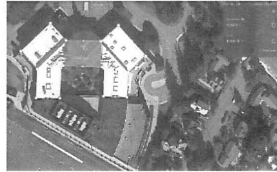
High School Roof-Building A
